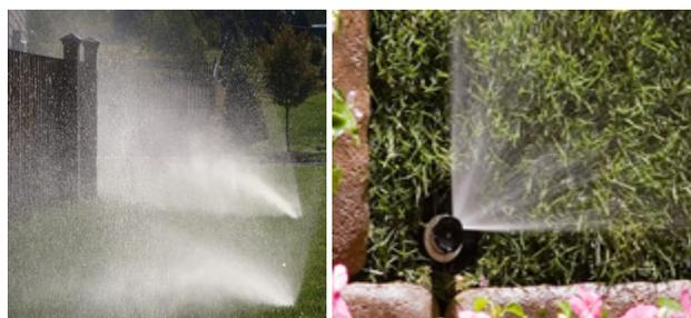
The system on the left is operating under too-high pressure (photo courtesy of Irrigation Association); the right photo shows correct pressure (photo courtesy of Rain Bird).
