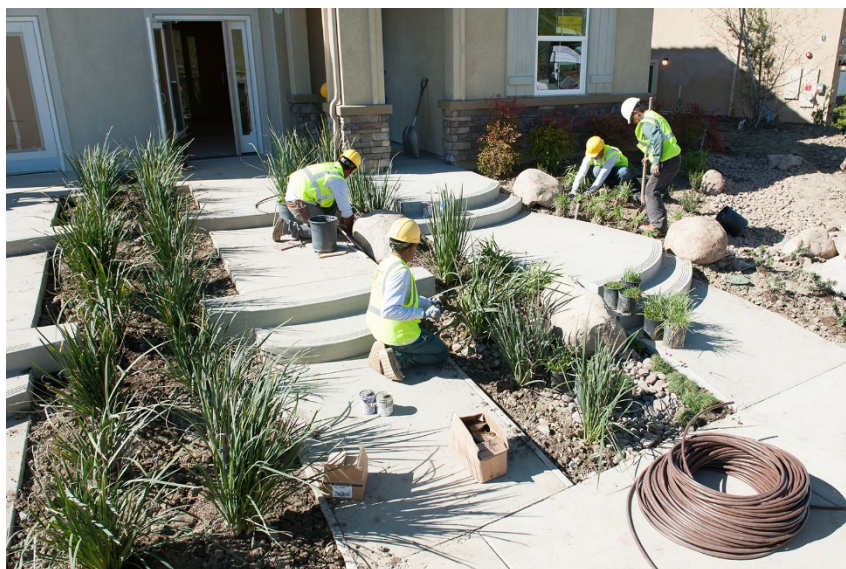
With the planting in place, landscape contractors begin to install dripline irrigation that will water plants at their rootball, eliminating overspray. (KB Home Rancho Santalina Community in San Marcos, California)
