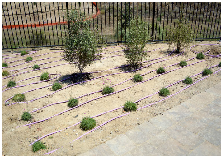
Dripline irrigation in a shrub planter bed. Water is delivered at the soil line to eliminate overspray and water runoff. Purple driplines denote the use of greywater for the irrigation system. (KB Home Sea Cliff Community in San Diego, California)
