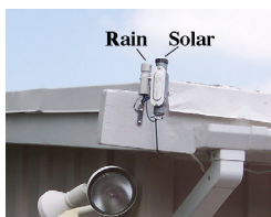
Sensors mounted on roof.
