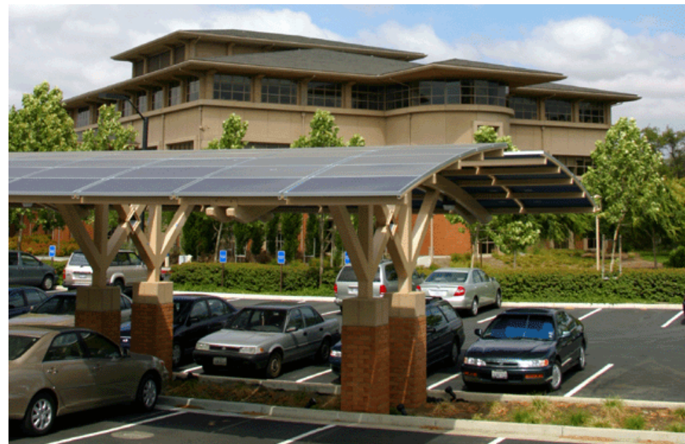
Solar carport in Headquarters parking lot
