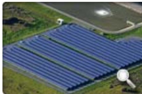
622kW Sewage Commission Oroville Region, CA 2003
