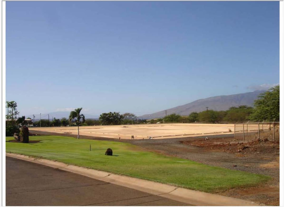
Onsite Covered Effluent Storage Pond
