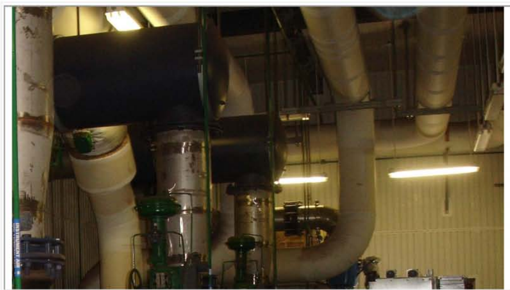
Indoor T12 Fluorescent Lighting
