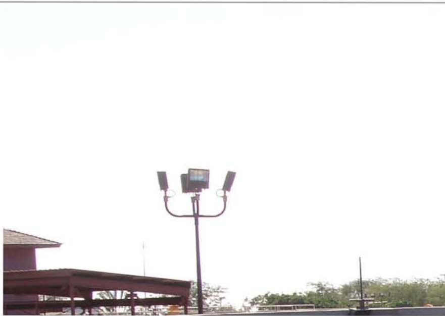
Outdoor Site Lighting
