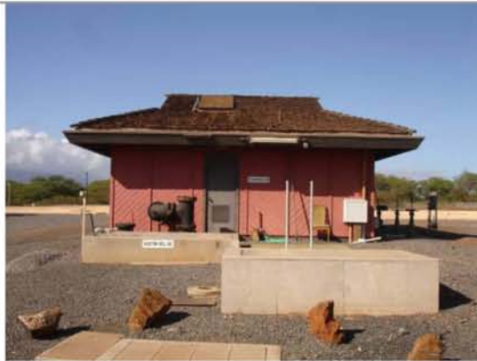
Effluent Pumping Station
