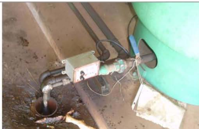
Sites Existing Air Condensate Drains – Timer Based Traps
