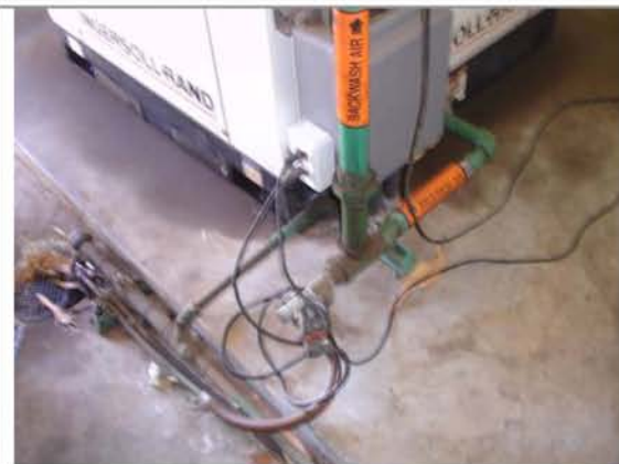
Sites Existing Air Condensate Drains – Timer Based Traps
