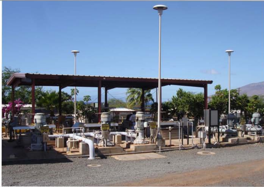
Outdoor Site Lighting
