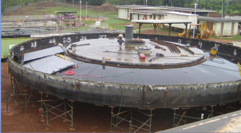
New wastewater treatment plant digester
