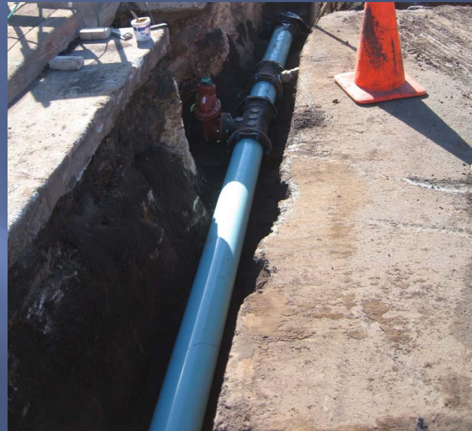
Waterline Replacements: Business Case required!
