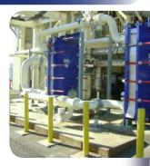
with two plate and frame heat exchangers. While each exchanger is sized to handle the cogeneration heat wasting requirements, a second unit was installed to provide redundancy for system maintenance. In addition, a larger drain valve was installed that reduces the time needed to drain and service the system from hours to minutes.
