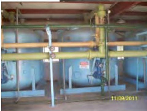
Green Sand Filter Tanks
