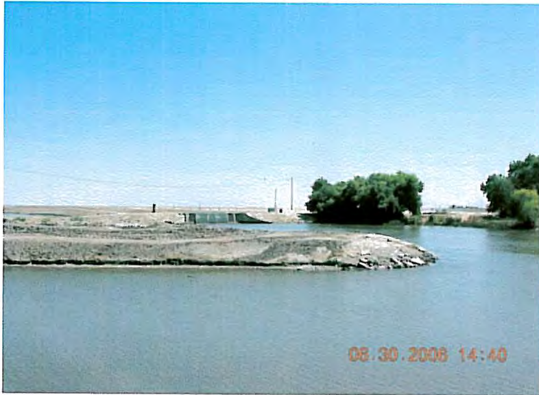
Kings River Canal south of structure on Kings River at Empire Weir No. 2.
