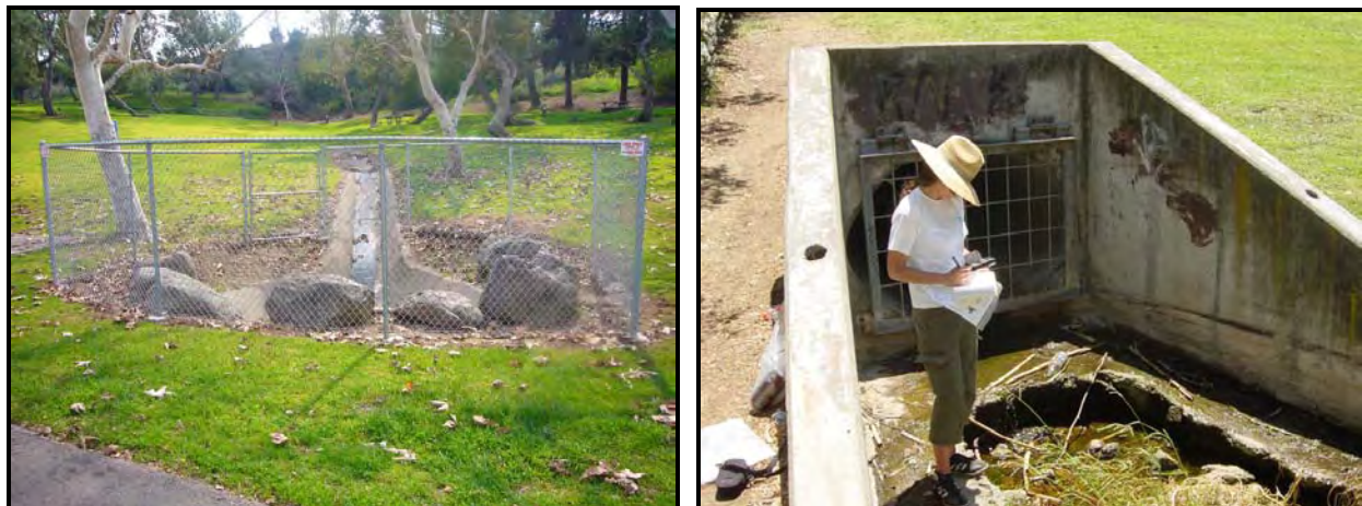
Figure 10-6. Storm Drain Discharges to Puddingstone Reservoir
