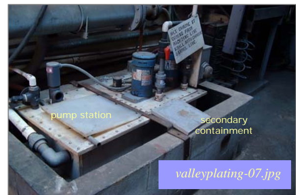
Photo #6: Pump Station for Chrome-Bearing Rinses Taken By: Greg V. Arthur Date: 09/09/08
