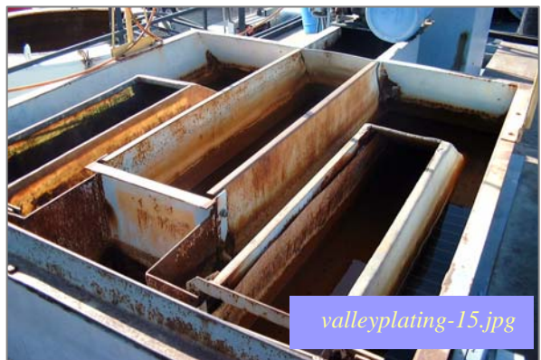
Photo #10: IWTP - Top of the Lamella Clarifier Taken By: Greg V. Arthur Date: 09/09/08
