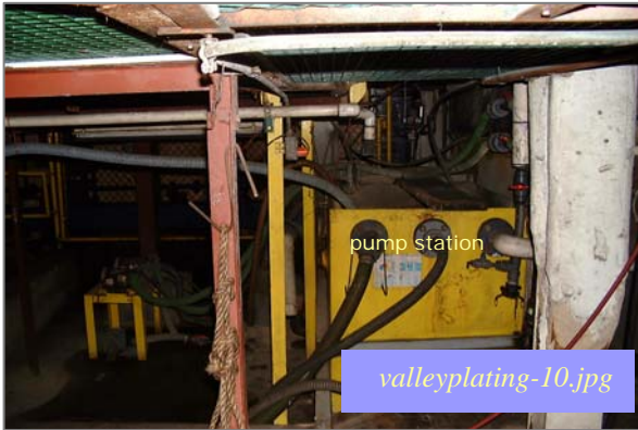
Photo #7: Lines E / F - Pump Station for Rinses Taken By: Greg V. Arthur Date: 09/09/08
