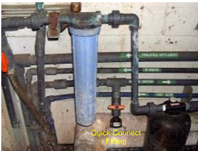
Photo No. 3 – Feeder Pipeline
