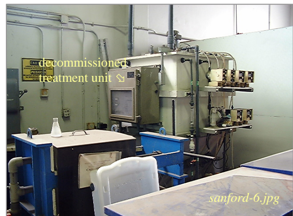
Photo: Decommissioned Treatment Unit Taken By: Greg V. Arthur Date: 04/04/06
