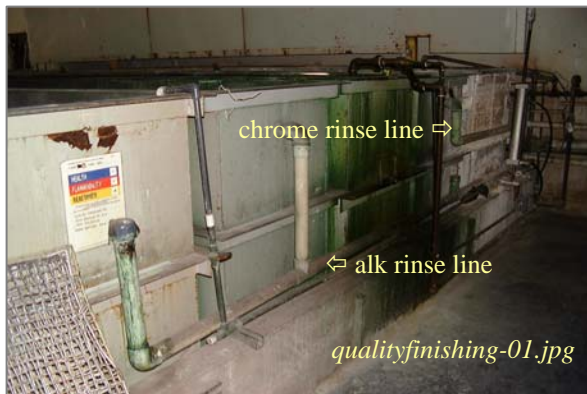
Photo #1: Conversion Coating Line Taken By: Greg V. Arthur Date: 09/09/08
