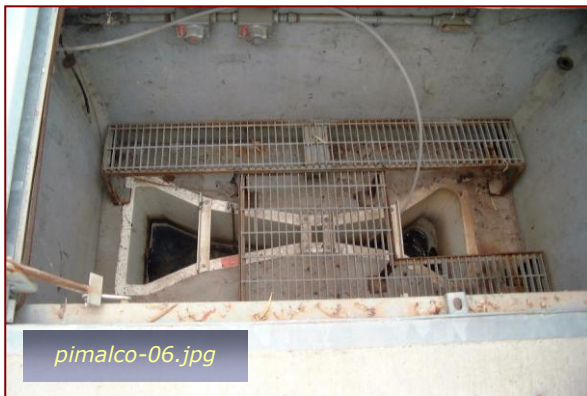
Photo #5: Final Discharge Point (IWD-19) Taken By: Greg V. Arthur Date: 08/11/09
