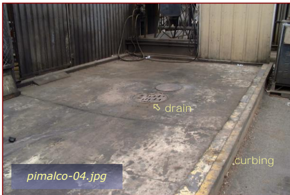
Photo #3: PSI Bldg – Steam Cleaning Pad Taken By: Greg V. Arthur Date: 08/11/09
