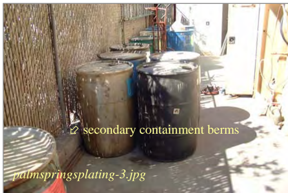
Photo: Drum Storage Area with 2 o Containment Taken By: Greg V. Arthur Date: 10/08/07
