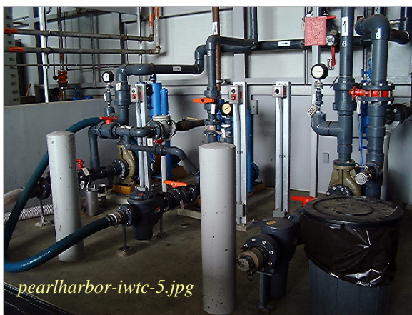
Photo: IWTC - Receiving Bay Taken By: Greg V. Arthur Date: 04/10/06
