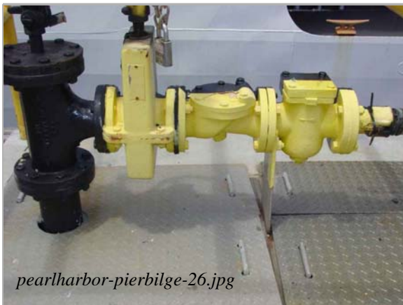
Photo: Pierside - Bilge Oily Wastewater Sewer Taken By: Julie Murioka, Navy Region Date: 04/12/06
