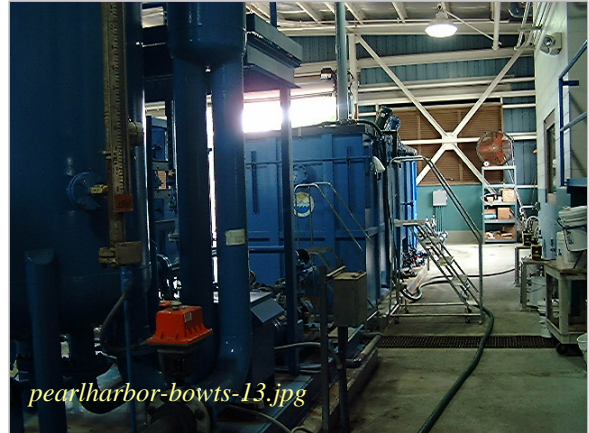
pearlharbor-bowts-13.jpg Photo: BOWTS - Treatment Unit B Taken By: Greg V. Arthur Date: 04/10/06
