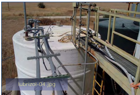
Photo #3: IWTP - 'Grey' Water Inlet Surge Tank Taken By: Greg V. Arthur Date: 08/10/11
