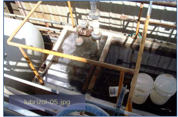
Photo #2: IWTP - Gravity Thickening Tank Taken By: Greg V. Arthur Date: 08/10/11
