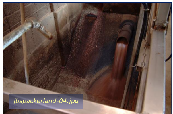
Photo #4: IWTP Influent Raw Wet Pit Taken By: Greg V. Arthur Date: 08/14/09
