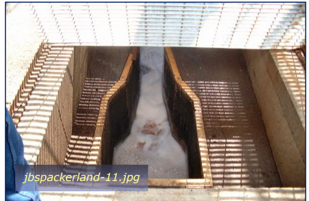
Photo #10: IWTP Effluent Flume (IWD-JBS1) Taken By: Greg V. Arthur Date: 08/14/09
