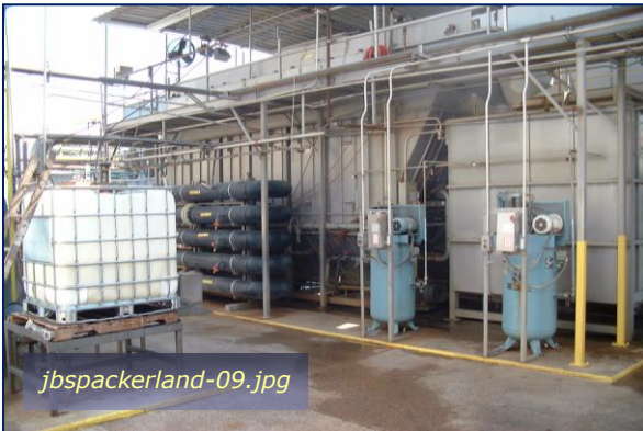
Photo #9: IWTP Induced Air Flotation (sideview) Taken By: Greg V. Arthur Date: 08/14/09
