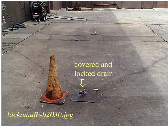
Photo: Bldg 2030 Washrack Covered Drain Taken By: Greg V. Arthur Date: 04/11/06
