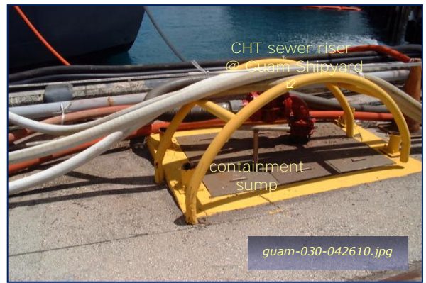
Photo #3-8: November Wharf CHT Sewer Riser Taken By: Greg V. Arthur Date: 04/26/10
