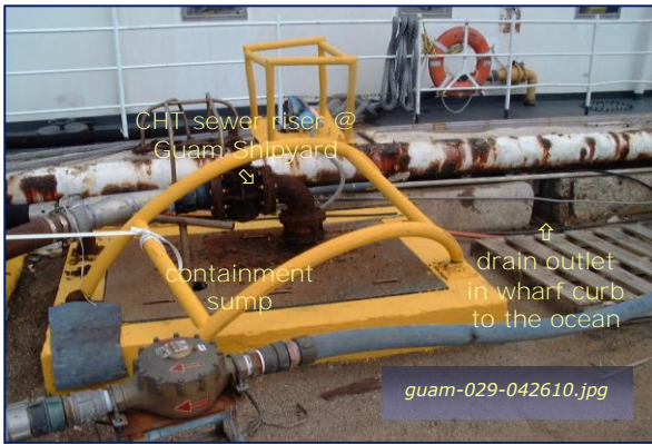
Photo #3-7: Oscar Wharf CHT Sewer Riser Taken By: Greg V. Arthur Date: 04/26/10
