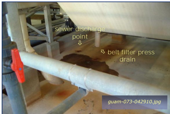
Photo #4-17: Fena WTP – Belt Filtrate Discharge Taken By: Greg V. Arthur Date: 04/29/10
