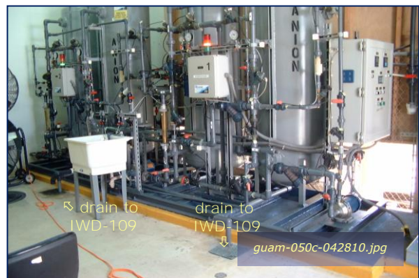
Photo #4-28: Bldg 4907 Demin Plant - IX Unit Taken By: Greg V. Arthur Date: 04/28/10
