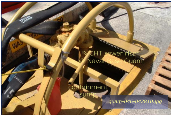
Photo #3-9: Sierra Wharf CHT Sewer Riser Taken By: Greg V. Arthur Date: 04/28/10
