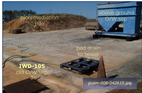
Photo #4-18: DRMO Haz Waste Facility - Pad Taken By: Greg V. Arthur Date: 04/26/10
