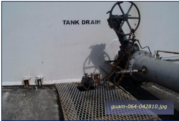
Photo #4-13: FISC Fuel Farm – Tank Bottom Draw Taken By: Greg V. Arthur Date: 04/28/10
