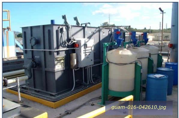
Photo #4-4: Victor Wharf BOTWS – Chem Treat Unit Taken By: Greg V. Arthur Date: 04/26/10
