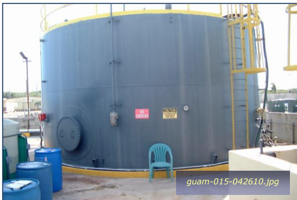
Photo #4-3: Victor Wharf BOWTS – 50kgal EQ Tank Taken By: Greg V. Arthur Date: 04/26/10
