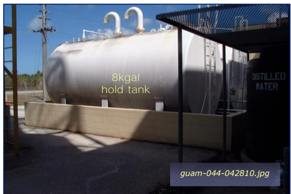
Photo #4-24: Bldg 307 Orote Power Plant – 8K Hold Taken By: Greg V. Arthur Date: 04/28/10
