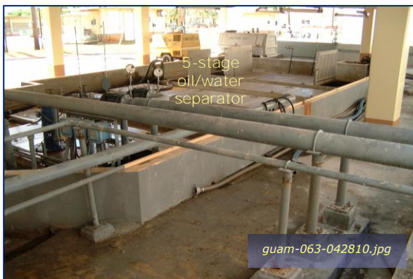
Photo #4-11: FISC Fuel Farm - O/W Gravity Sep Taken By: Greg V. Arthur Date: 04/28/10
