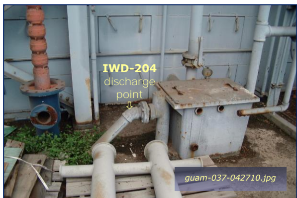
Photo #5-6: Bldg 27 Paint Shop - Sewer Connection Taken By: Greg V. Arthur Date: 04/27/10
