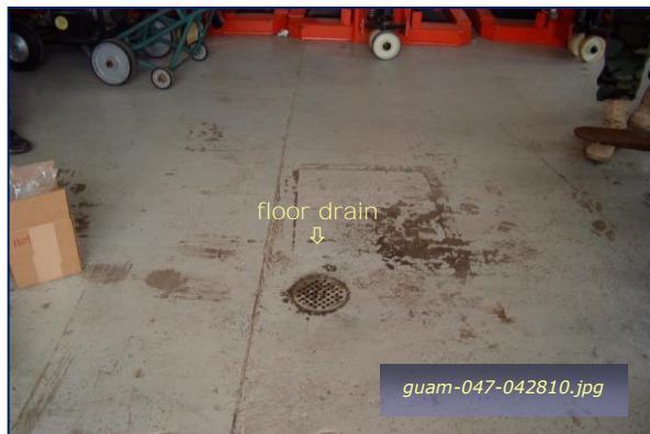
Photo #4-36: Bldg 2113 EOD – Example Floor Drain Taken By: Greg V. Arthur Date: 04/28/10
