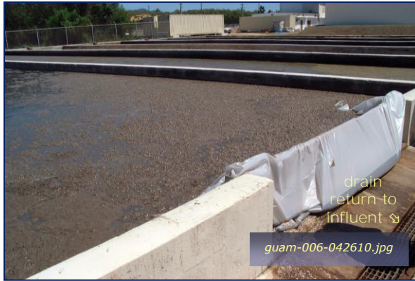
Photo #3-5: Apra Harbor WWTP - Sludge Drying Taken By: Greg V. Arthur Date: 04/26/10
