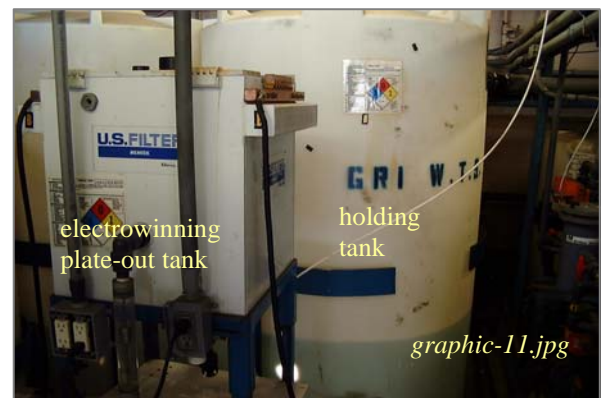
Photo #6: IWT Unit B - Holding and Plate-Out Taken By: Greg V. Arthur Date: 09/09/08
