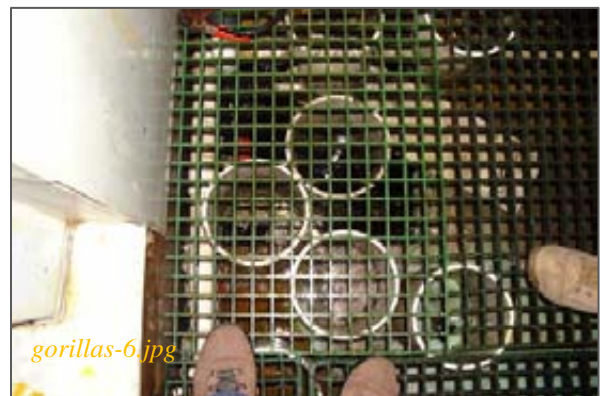
Photo #4: Inlet sump for chrome-bearing flows Taken By: Greg V. Arthur Date: 09/11/08
