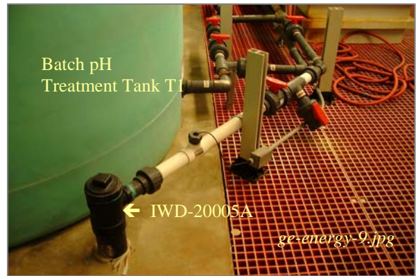
Photo: Final pH Adjustment and Sample Point Taken By: Greg V. Arthur Date: 11/27/07
