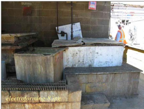
Photo: Stripping Area "D" with 2° Containment Taken By: Anna Yen Date: 08/28/07
