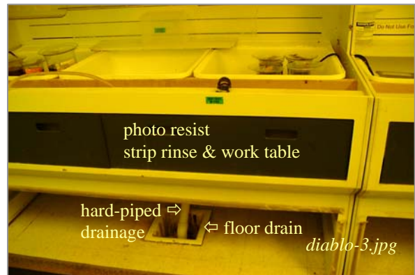
Photo #1: Photo Resist Work Table / Floor Drain Taken By: Greg V. Arthur Date: 11/27/07
