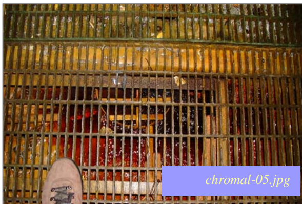
Photo #3: Closed-Loop Rinse Reuse Floor Sump Taken By: Greg V. Arthur Date: 09/10/08
