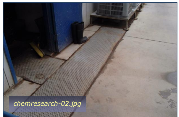
Photo #4: Collected Outdoor Drainage to IWTP Taken By: Greg V. Arthur Date: 08/13/09
