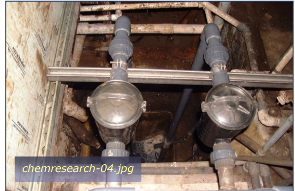
Photo #2: Cr-plating Ion Exchange Canisters Taken By: Greg V. Arthur Date: 08/13/09
