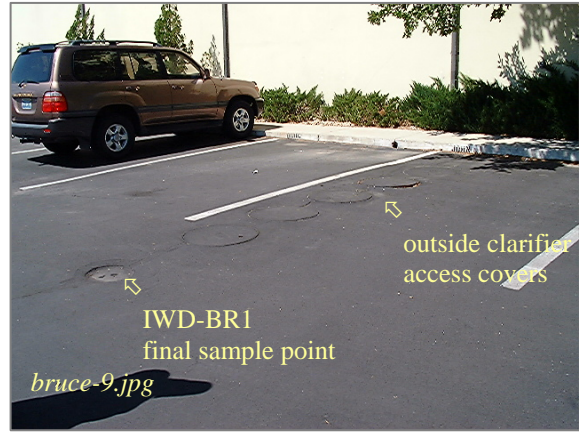
Photo: Location of Outside Clarifier Taken By: Greg V. Arthur Date: 07/20/06
