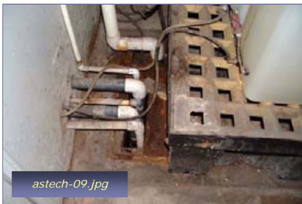
Photo #9: X-ray Developer Rinses into Sump Taken By: Greg V. Arthur Date: 09/12/08
