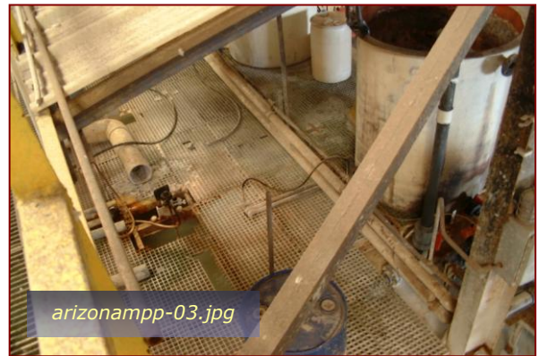
Photo #2: 2° Containment Pit Taken By: Greg V. Arthur Date: 08/12/09
