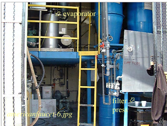
Photo: Filter Press and Evaporator Room Taken By: Greg V. Arthur Date: 05/03/07
