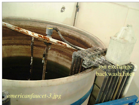
Photo: Batch Treatment Tank for IX Backwash Taken By: Greg V. Arthur Date: 05/03/07
