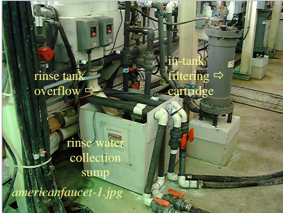
Photo: Rinse Water Collection and Filter Cartridge Taken By: Greg V. Arthur Date: 05/03/07
