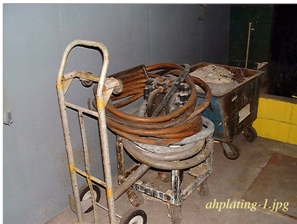
Photo: Portable pump and hosing Taken By: Greg V. Arthur Date: 09/06/06
