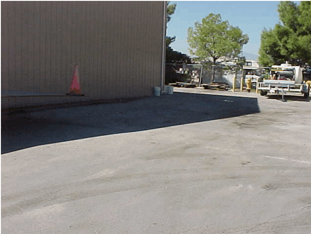
Photo 5. Fleet (primary) facility: Truck wash area is outside, uncontained, uncovered.
