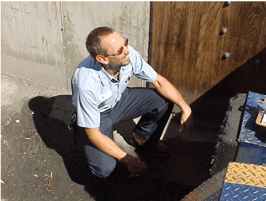
Photo 4. Mr. Palsgrove inspecting loading dock and dead sump for collection of storm water.
