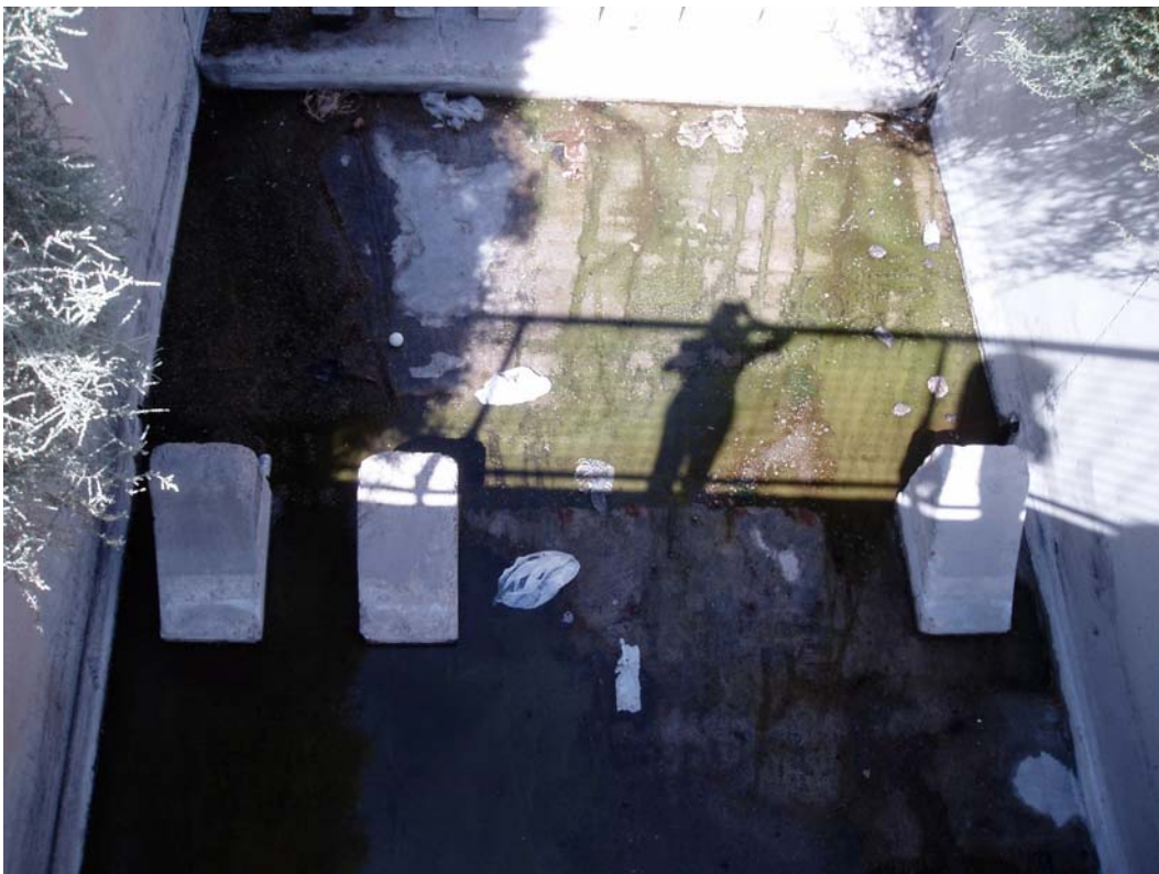
Photo 12. Bottom of Union Pacific Railroad Channel.
