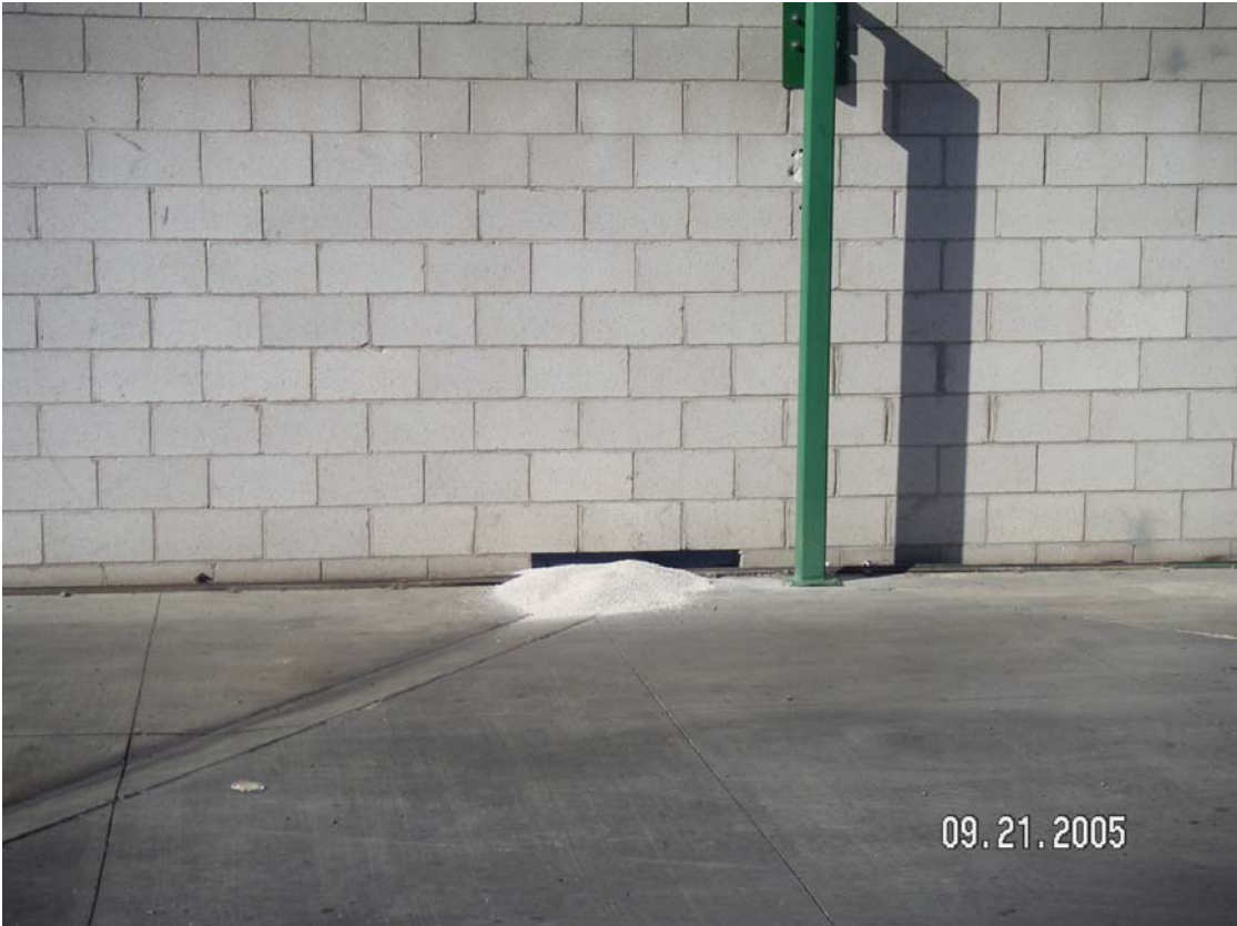
Photo 5. Absorbent material at point of outflow from yard.
