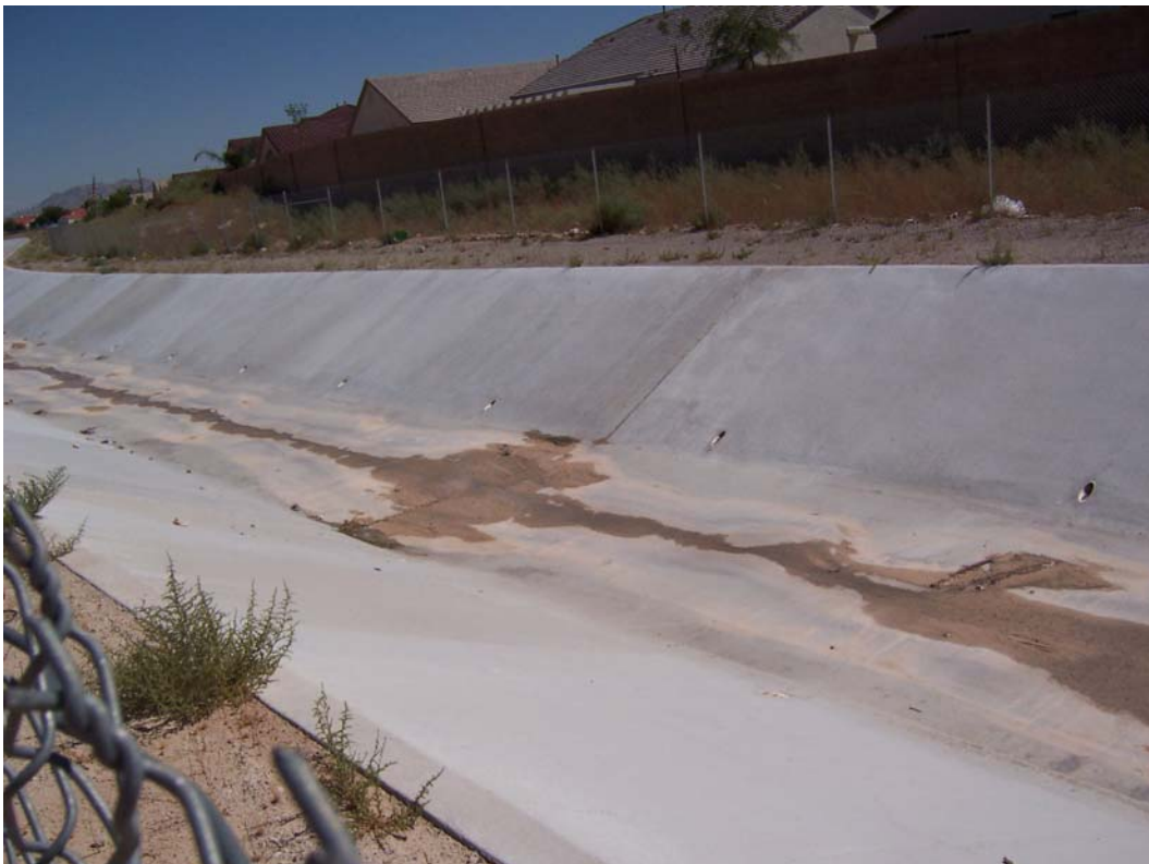
Photo 2. Wash adjacent to the construction site. Wash appears to contain sediment that may have come from the site.
