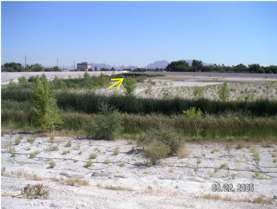
Photo 9. Meadows Detention Basin - outlet area.
