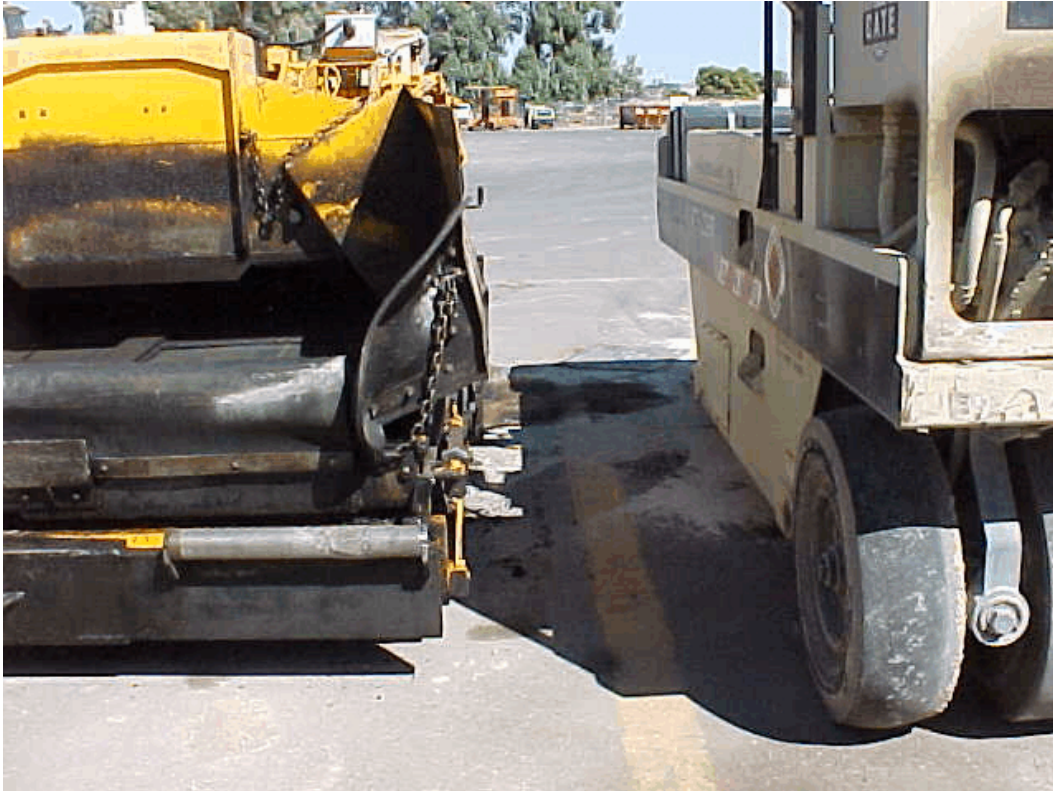
Photo 11. Fleet (secondary) facility: Truck and paving equipment parking area with spills/leakage staining on pavement.
