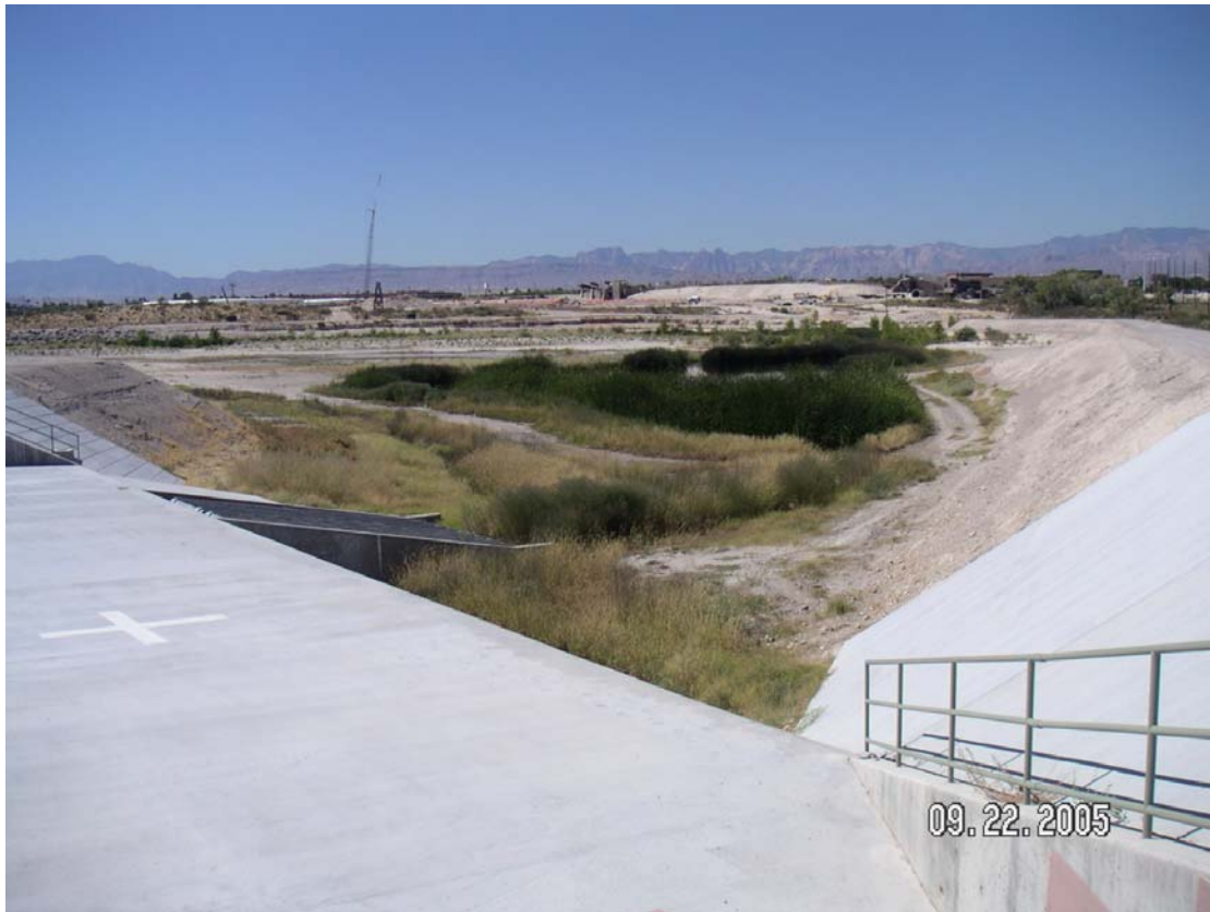
Photo 15. Meadows Detention Basin - grate at effluent from basin.
