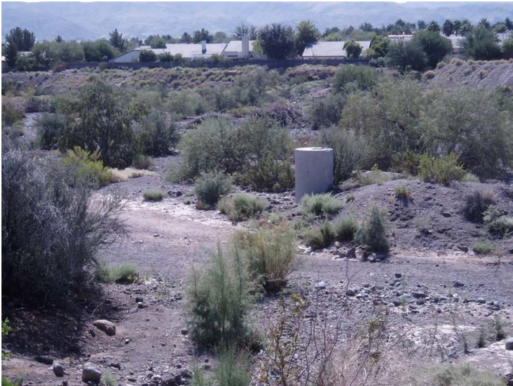
Photo 3. Project Green, elevated manhole in photo center.
