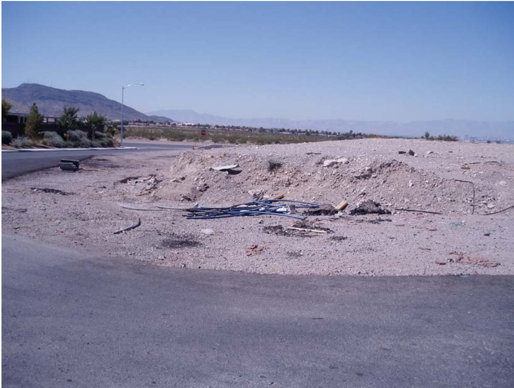
Photo 1. Debris at construction site entrance.
