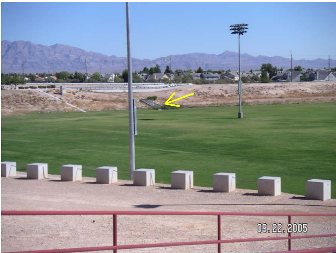
Photo 2. Gowan Detention Basin - outlet.
