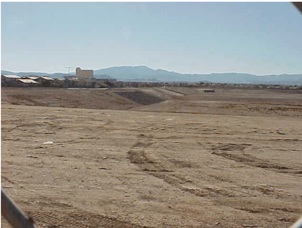
Photo 2. Southwest view of the detention basin from the east fence.
