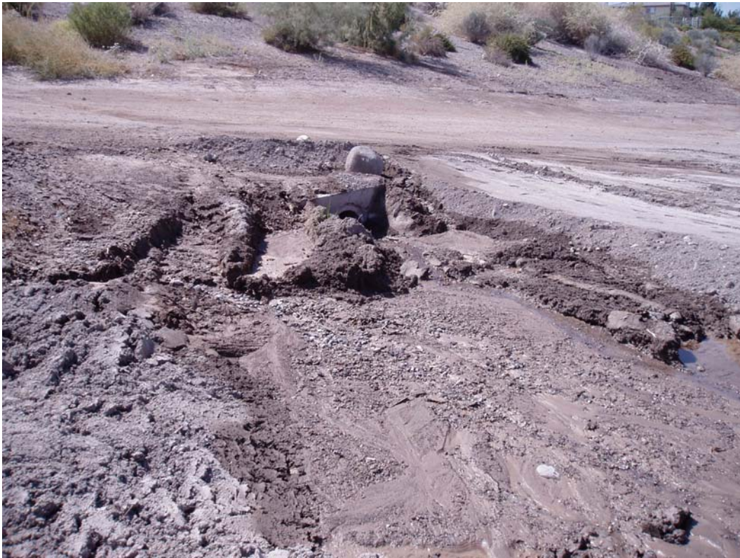
Photo 17. Outfall that discharges groundwater.
