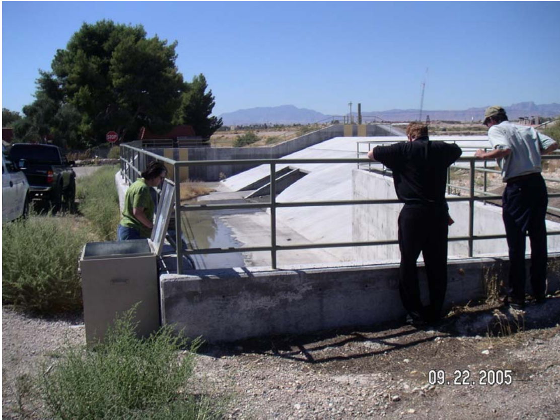
Photo 13. Meadows Detention Basin - effluent sampler and outfall.
