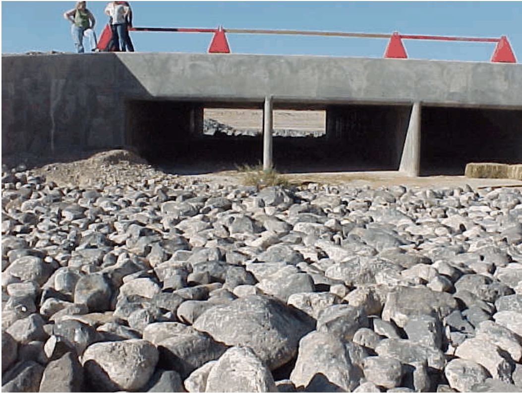
Photo 5. View of the wash passing under the street to the detention basin.
