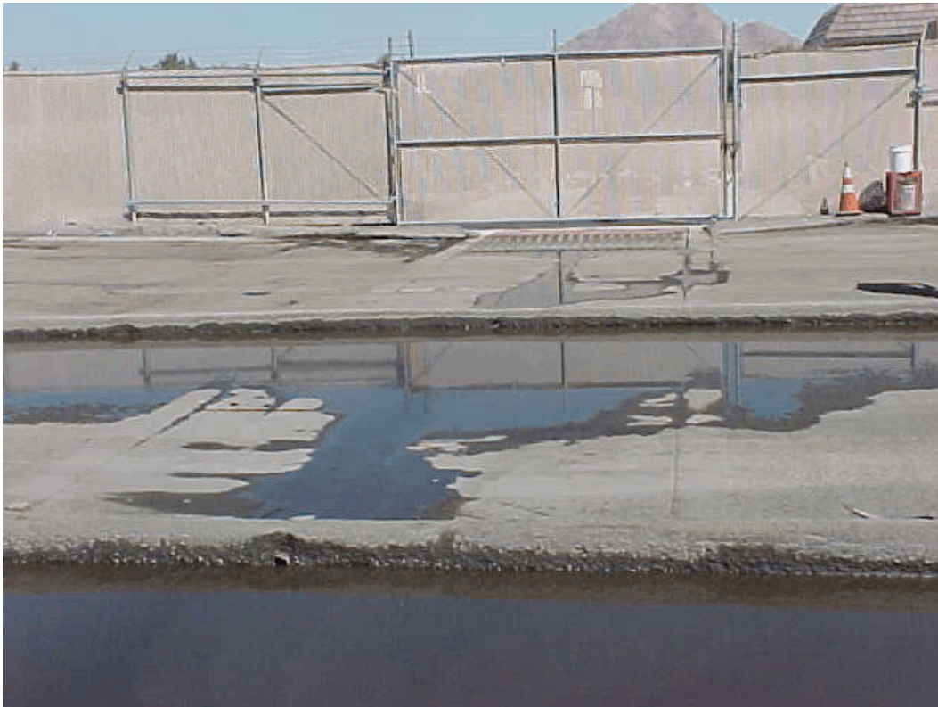
Photo 3. Sediment traps to collect soil and debris from street sweeper unloading.
