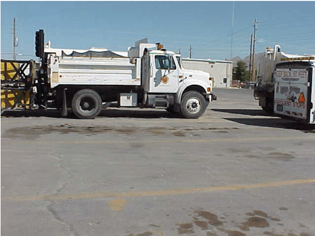
Photo 8. Fleet (primary) facility: Truck parking area with spills/leakage staining on pavement.
