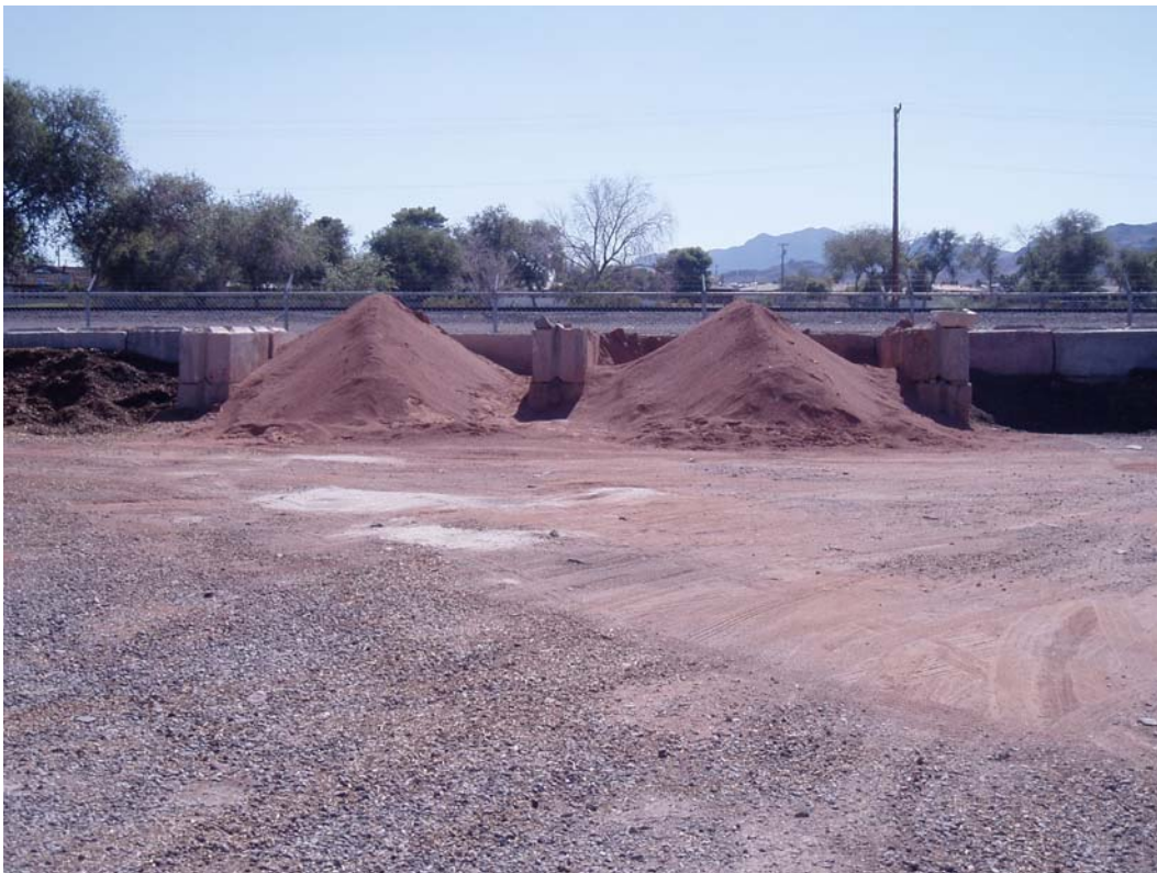
Photo 4. Sediment stockpiles. Grade is downhill toward the street.
