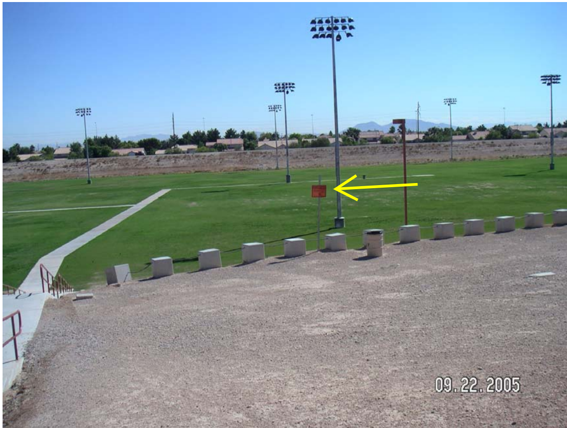
Photo 3. Gowan Detention Basin - signage.
