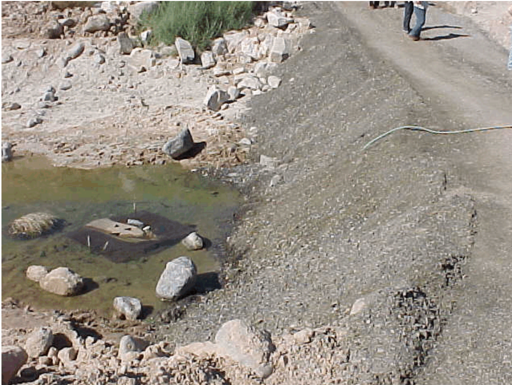
Photo 1. Diversion inlet (photo left) and earthen dam.
