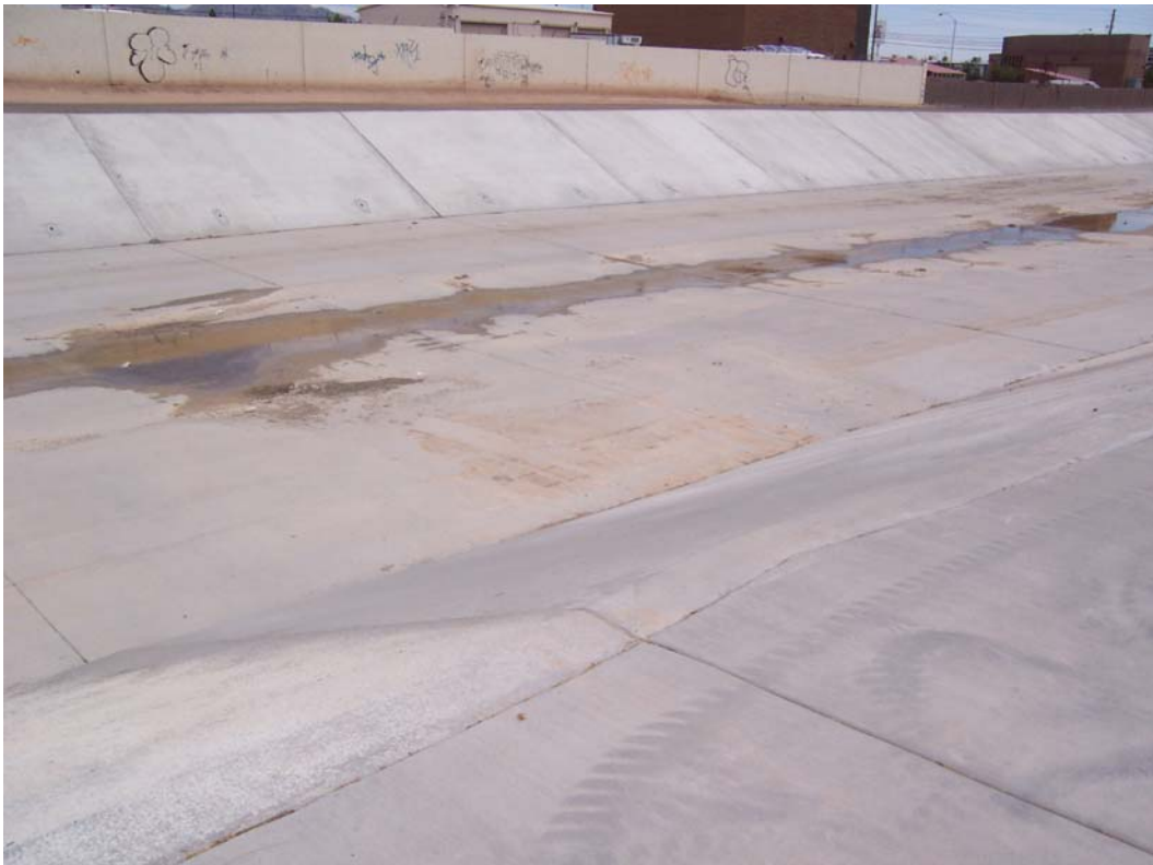
Photo 5. Portion of wash adjacent to the channel in Photo 4 where sediment appears to have entered the wash from the channel.
