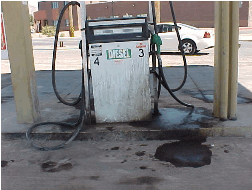
Photo 6. Spillage at fuel island.
