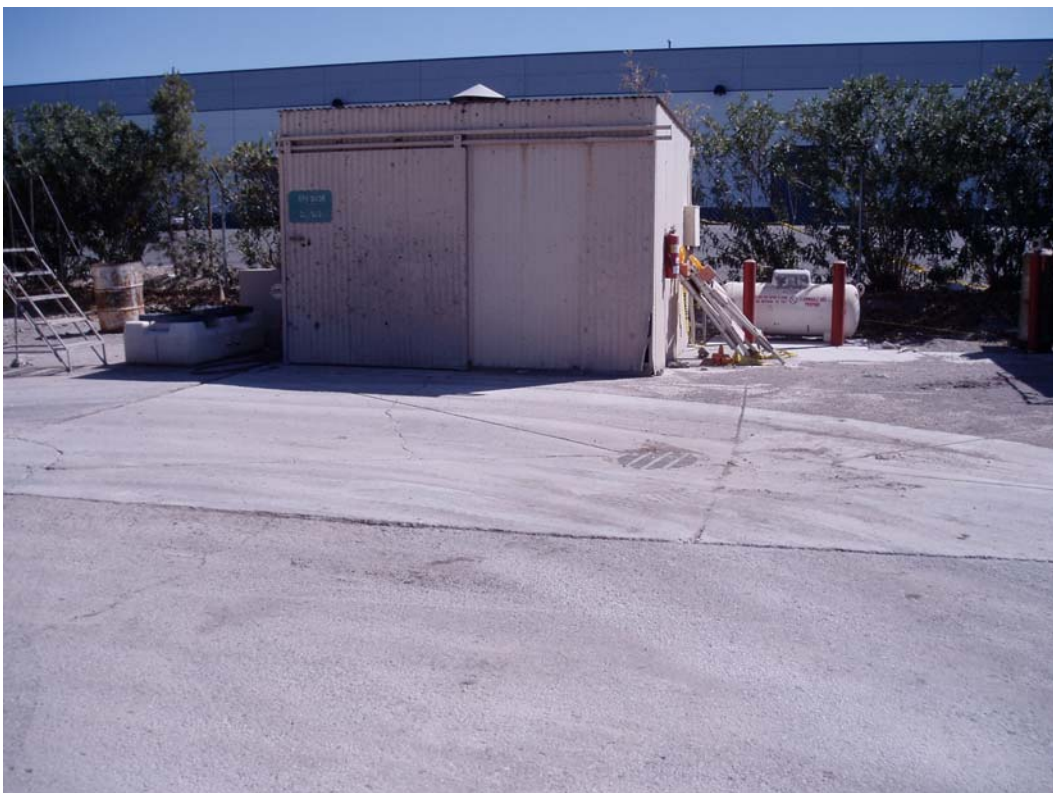
Photo 2. Car wash area. Drain flows to sanitary sewer.
