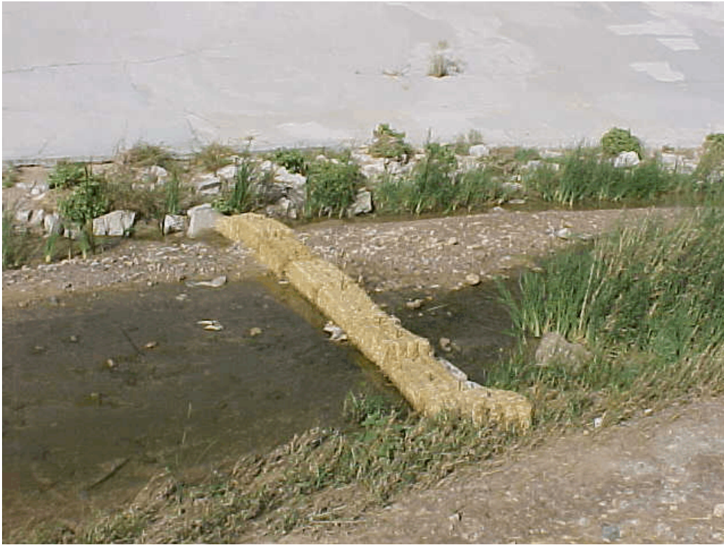
Photo 5. View of straw bale filter in Duck Creek Channel downstream from the construction area.
