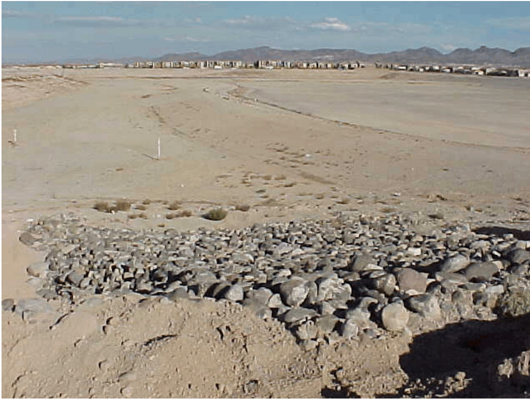
Photo 7. East view of detention basin.
