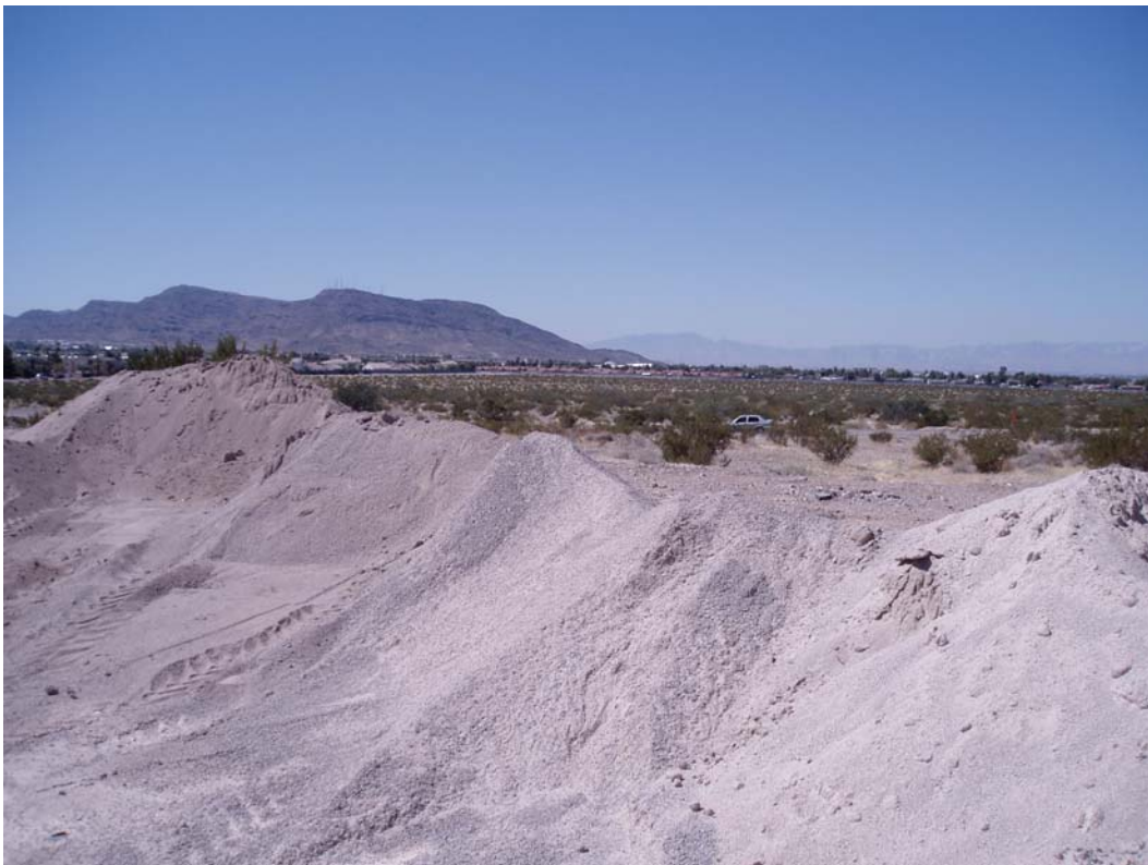
Photo 2. Sediment stockpiles. Note the ground slopes towards the road in the background.
