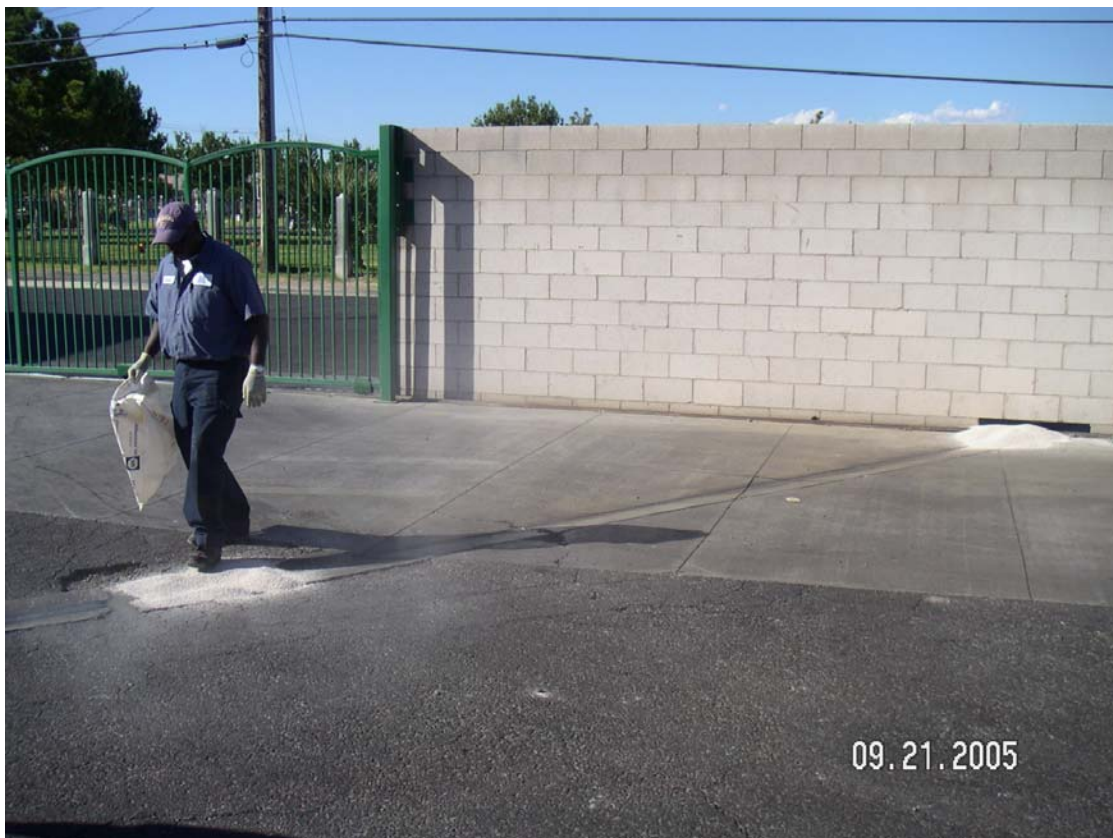
Photo 4. Worker spreading absorbent material.
