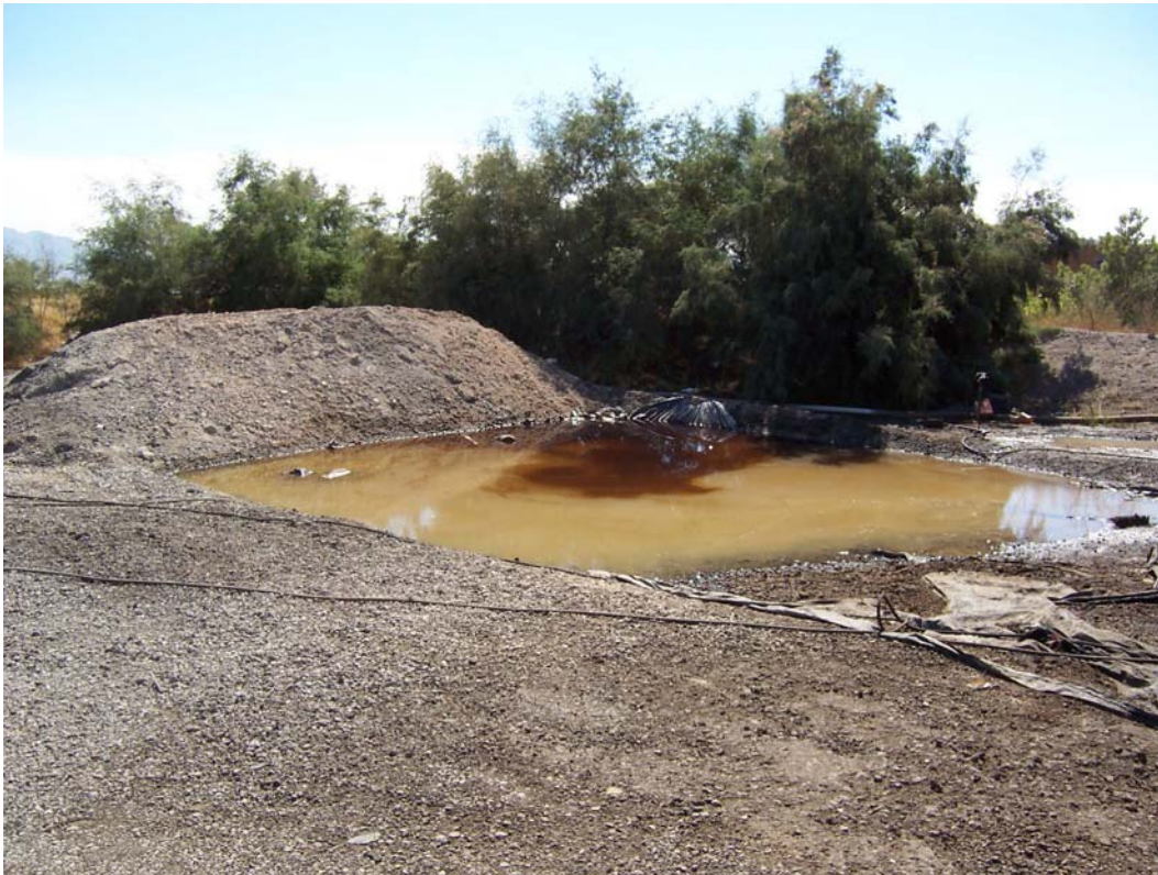
Photo 3. Temporary pit dug to contain wash water from equipment cleaning operation. Note floating oil on the surface of the water.
