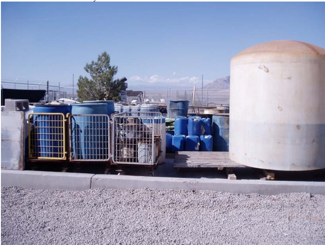
Photo 2. Bermed area for chemical storage.
