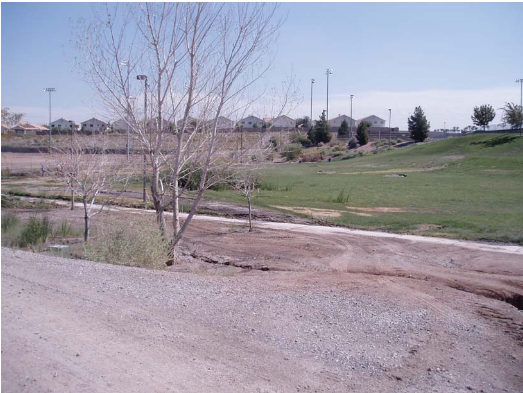
Photo 18. Detention basin/baseball field.
