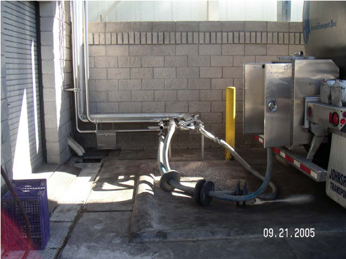
Photo 6. Tank truck off loading area.
