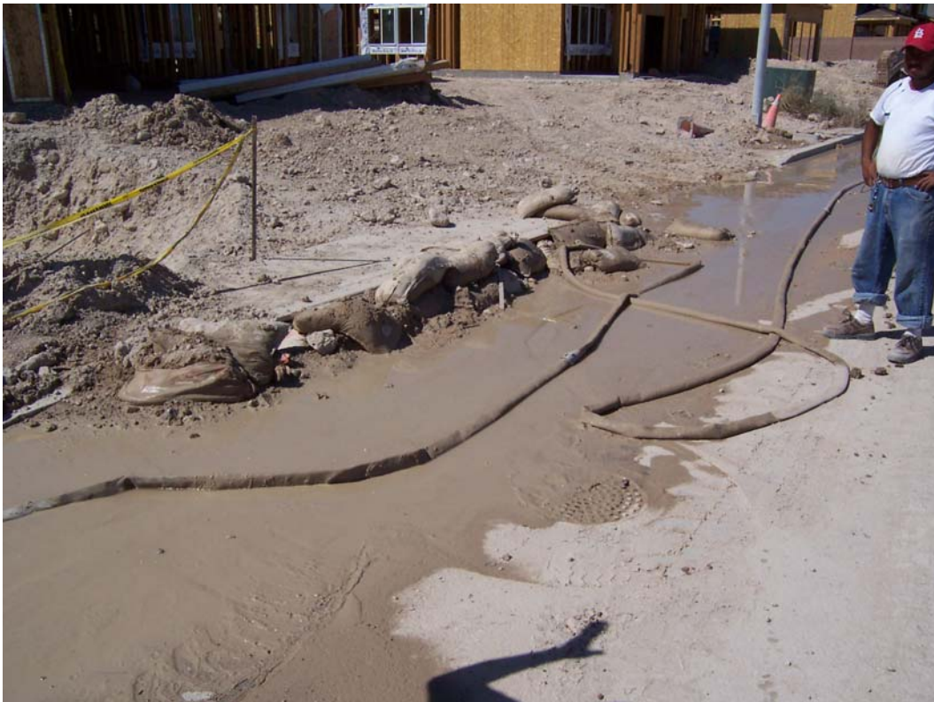
Photo 2. Storm inlet at the site. Sediment is also entering the storm sewer through the pick hole in the manhole in front of the inlet. Hose in the photo is the fire hose the site had been using to clean the street. Note poor condition of sand bags used for inlet protection and dirt extending past curb line.
