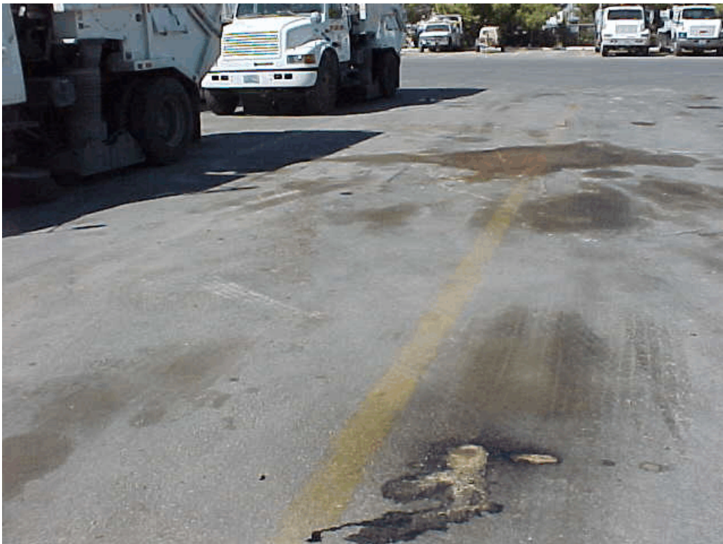
Photo 10. Fleet (primary) facility: Truck parking area with spills/leakage staining on pavement.
