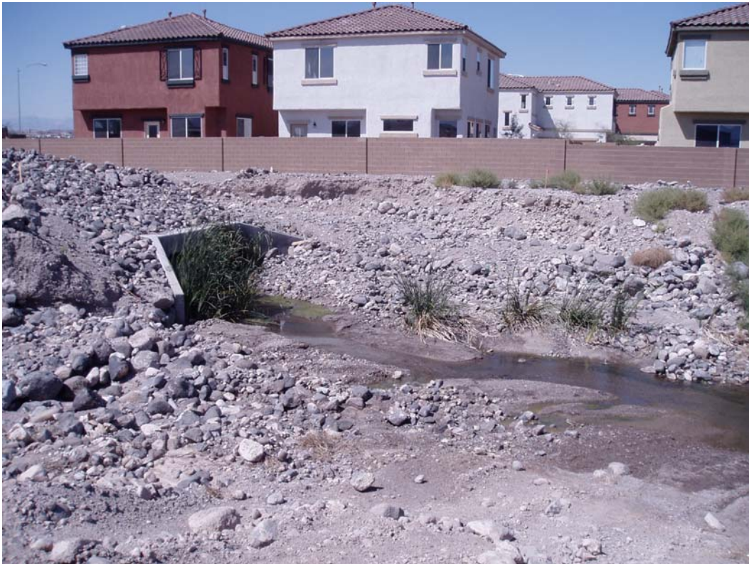
Photo 25. Outfall with flow.
