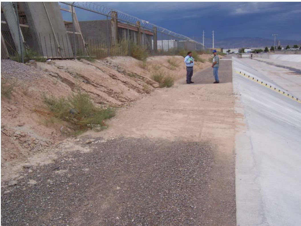
Photo 6. Area where soil erosion on the bank to the left of the wash appears to have entered the wash.
