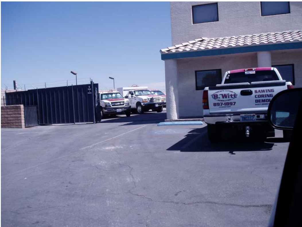
Photo 30. Parking lot source of discharge in Photo 29.
