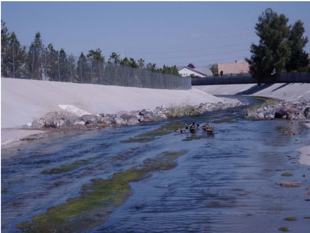
Photo 20. Bottom of channel.
