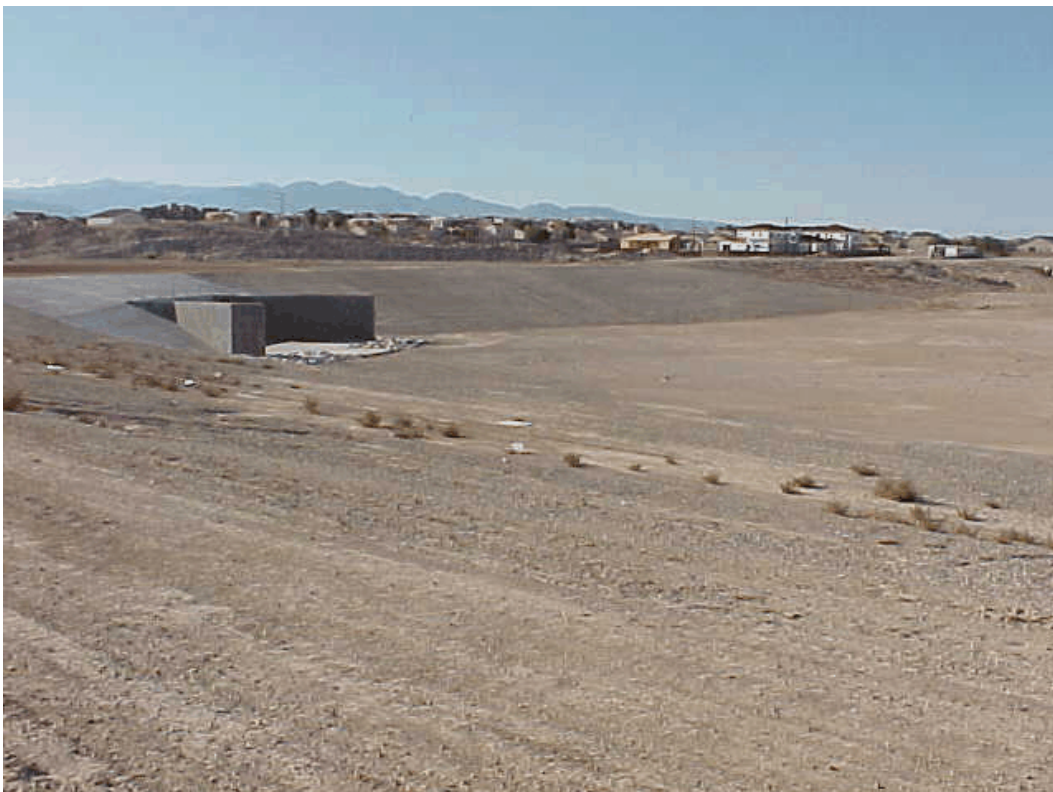
Photo 6. Inlet to detention basin at southwest corner.
