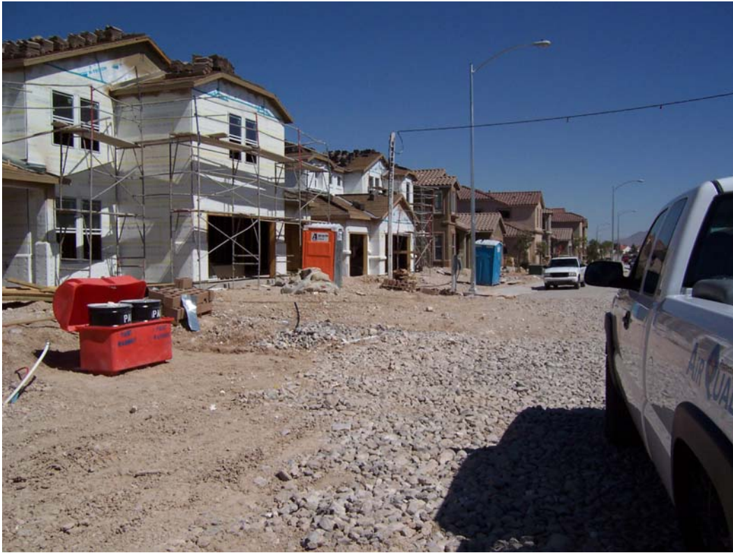
Photo 3. Note portable toilet (blue) in photo right center located immediately adjacent to the paved road upslope of inlets. Note also crush rock for trackout control located in front of pickup truck at photo right.
