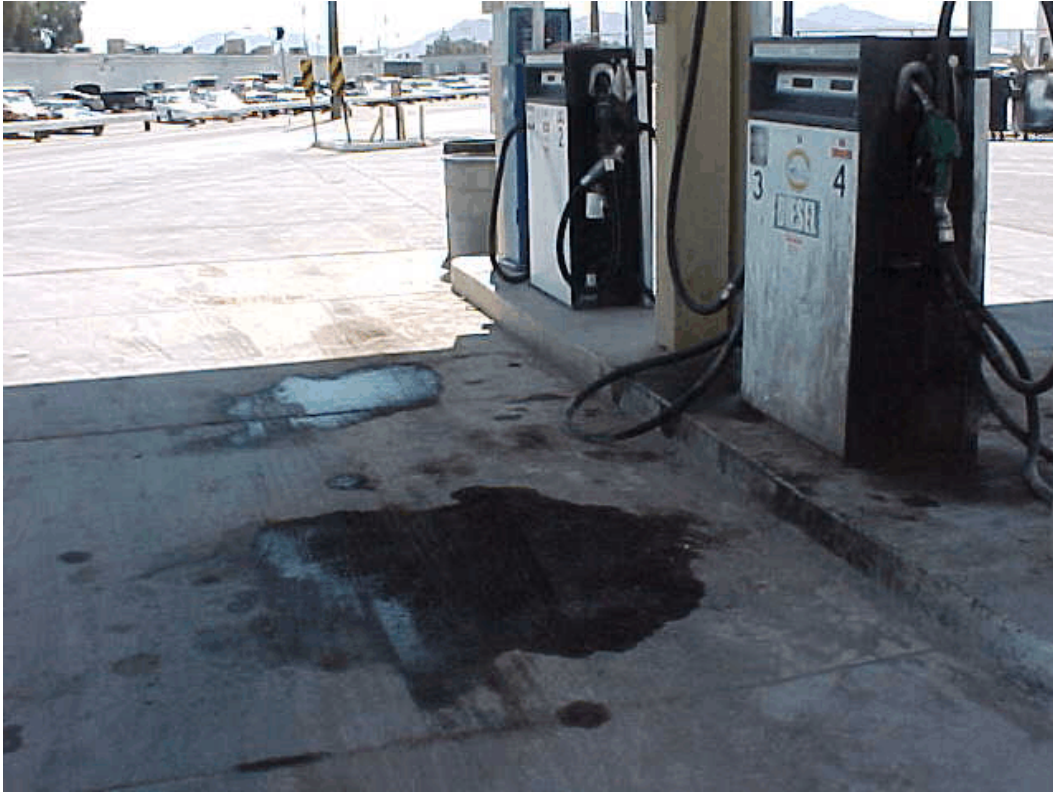
Photo 7. Spillage at fuel island.
