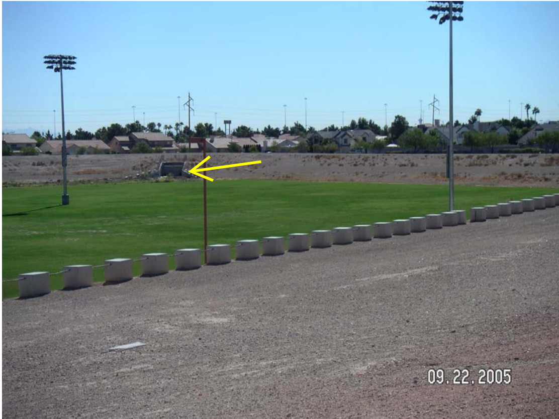
Photo 1. Gowan Detention Basin - inlet.
