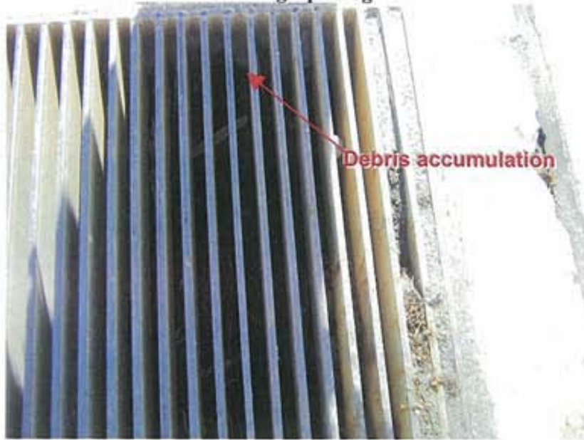
Photograph 23: At the location shown in Photographs 21 and 22, debris and/or tenant product had accumulated in the trench drain to nearly the top of the inlet grate
