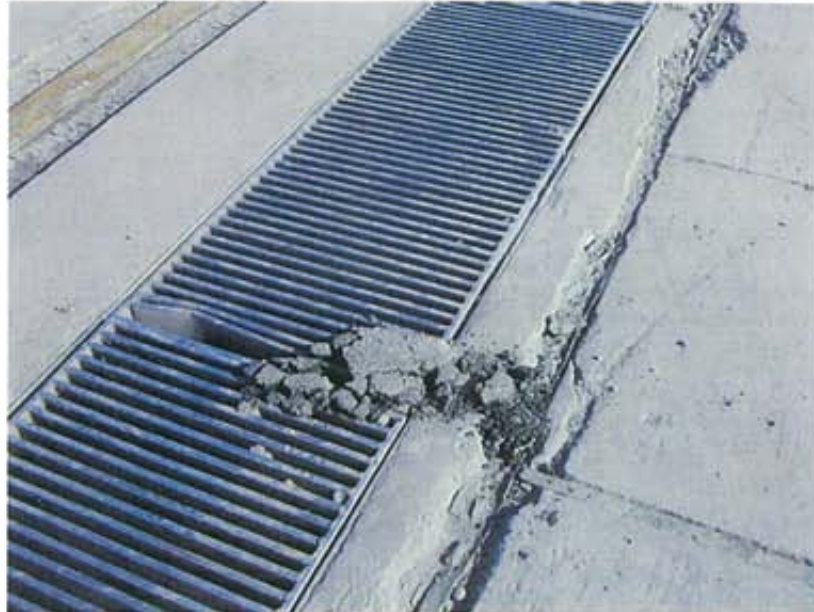
Photograph 12: View of location shown in Photograph 11
