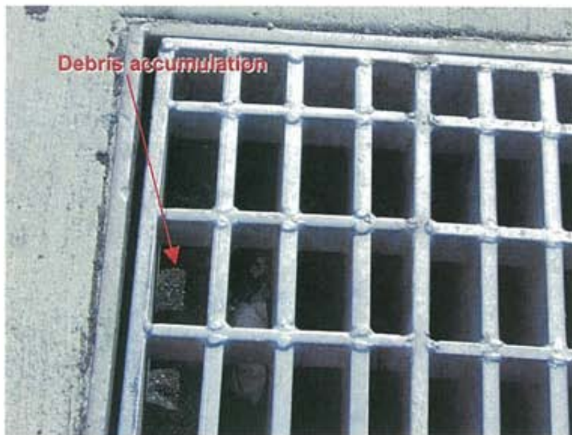
Photograph 20: View inside trench drain shown in Photograph 18
