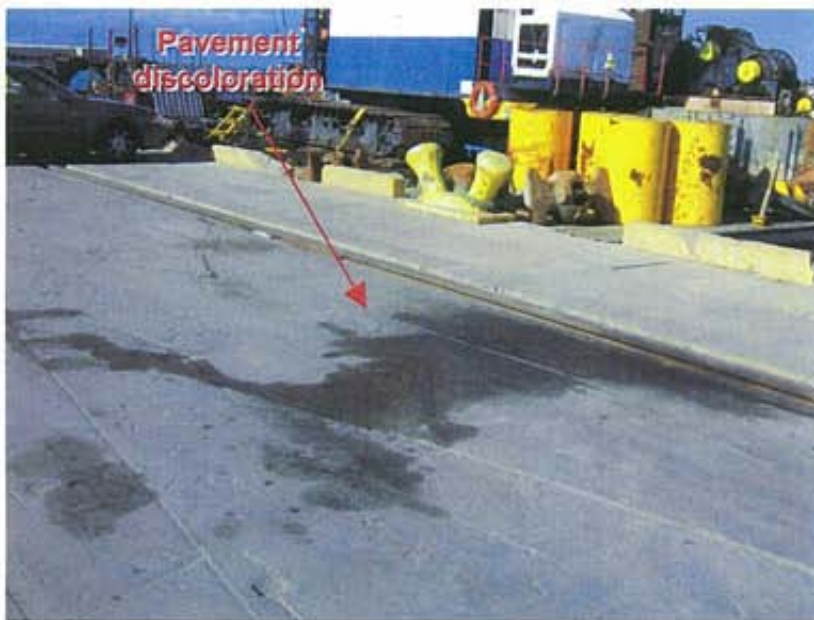
Photograph 14: View of Pavement discoloration and/or spill residues extending to the north of Photograph 13
