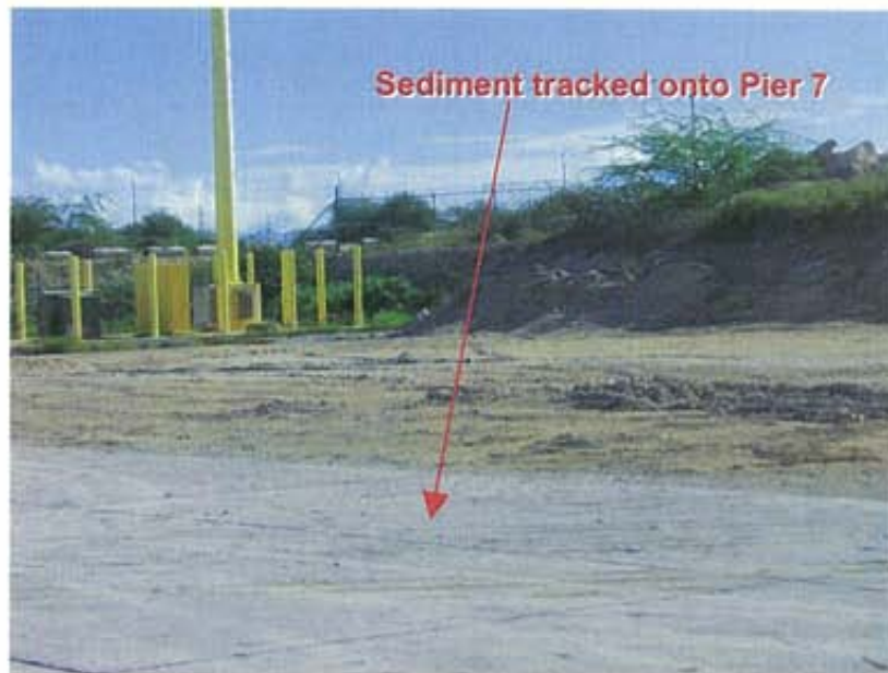
Photograph 8: Sediment had been tracked from area of lighting improvement disturbance onto the adjacent impervious pier surface
