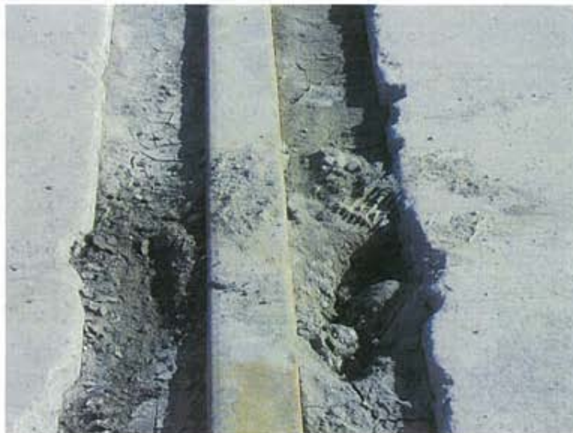
Photograph 10: Close-up view of accumulated pollutants showing potential for mobilization
