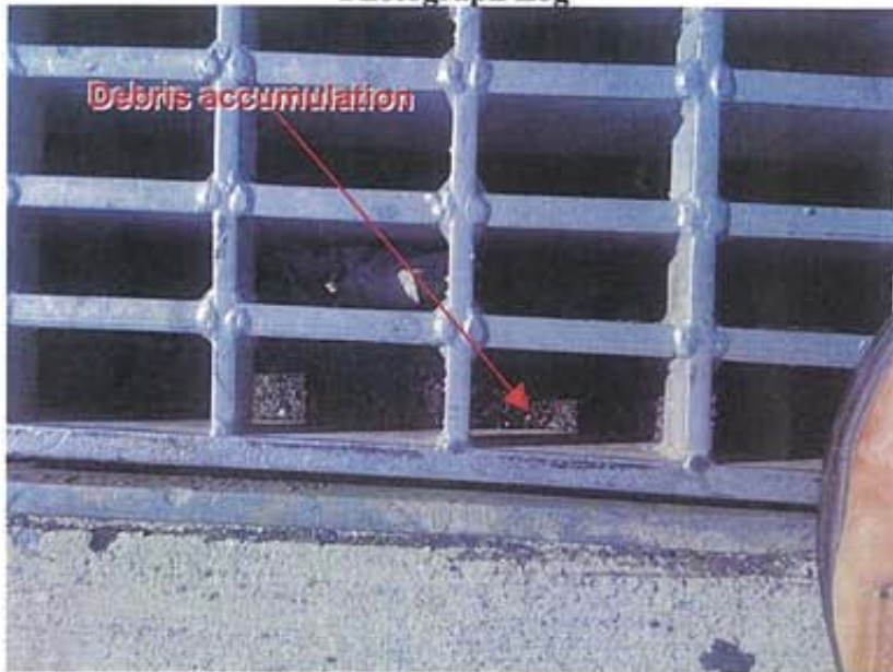
Photograph 19: View inside trench drain shown in Photograph 18
