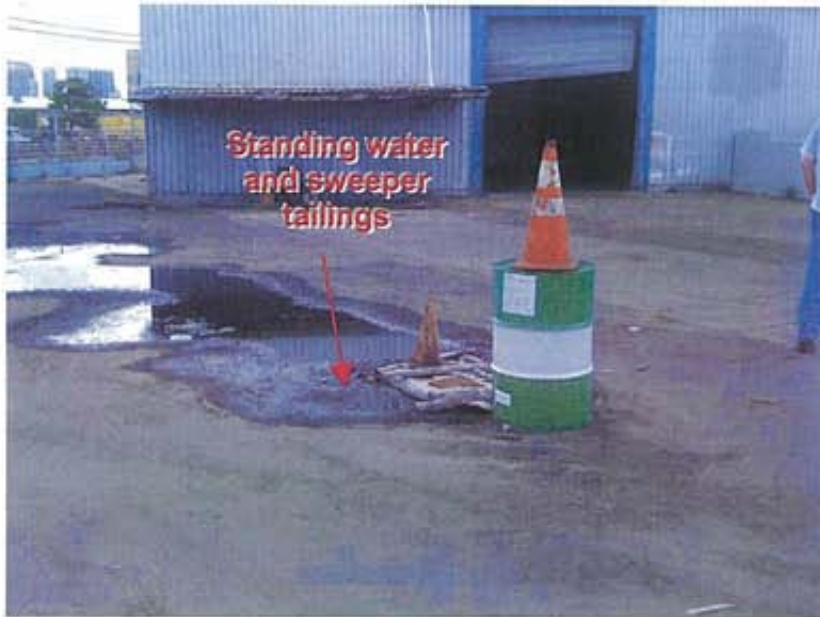
Photograph 3: Evidence of previous sweeper washout activity, including standing water and sweeper tailings near the storm drain inlet
