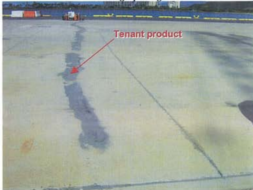
Photograph 21: At Piers 5 and 6 in Kalaeloa Barbers Point Harbor, tenant product had been spilled adjacent to a trench drain
