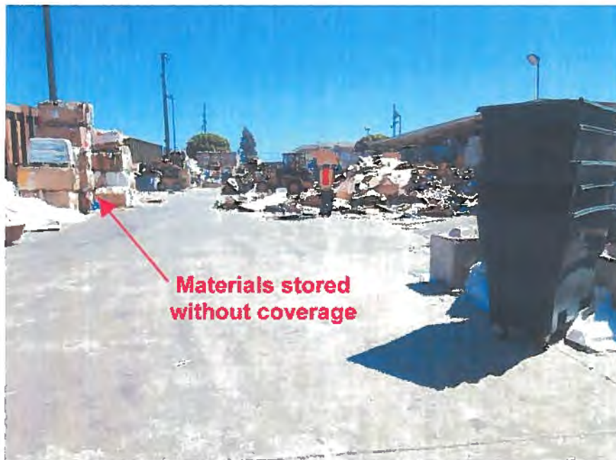
Photograph 1. Rincon Facility I/C Site Visit – View looking south of materials stored at the facility without coverage.
