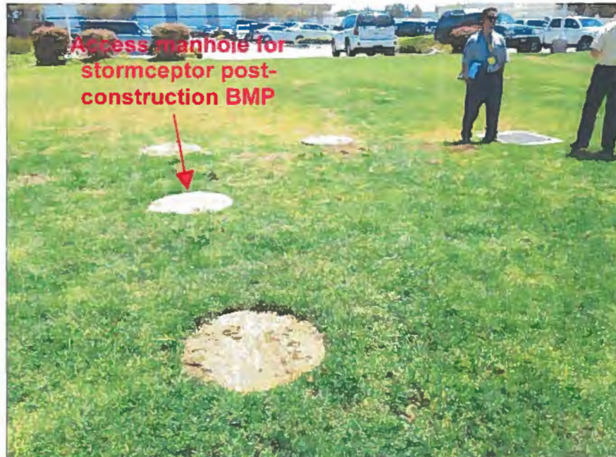
Photograph 5. PTI Facility I/C Site Visit – View of access manhole for stormceptor located on the north end of the facility.
