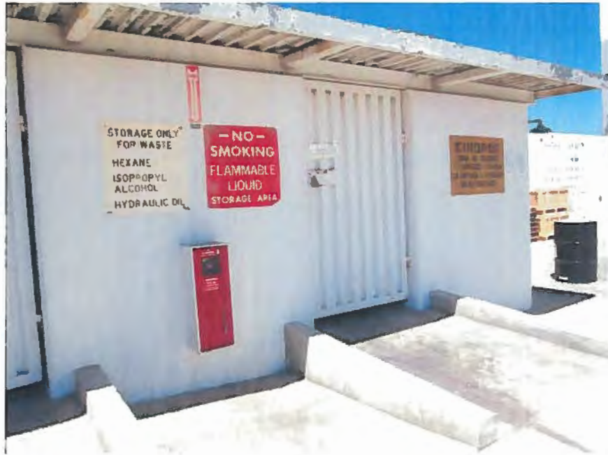
Photograph 3. PTI Facility I/C Site Visit – View of hazardous materials shed located on the northern side of the paved yard.
