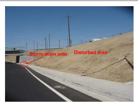
Photograph 3. View of disturbed slope where wattles were not present on the new embankments south of Hageman Road.
