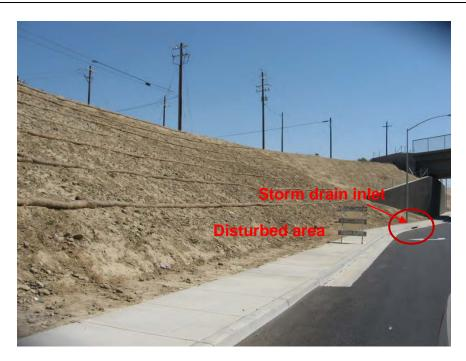
Photograph 1. View of wattles which had been installed on several new embankments surrounding the railroad overpass. Note that erosion from the lower level would be discharged to the storm drain inlet because protection had been removed.
