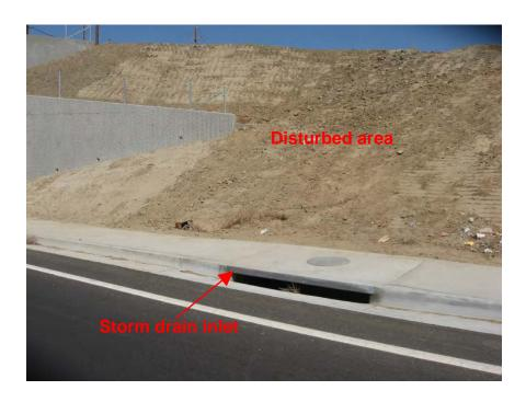
Photograph 4. View of storm drain inlet without BMPs for inlet protection. Storm drain inlets surrounding the project area were found to be unprotected.
