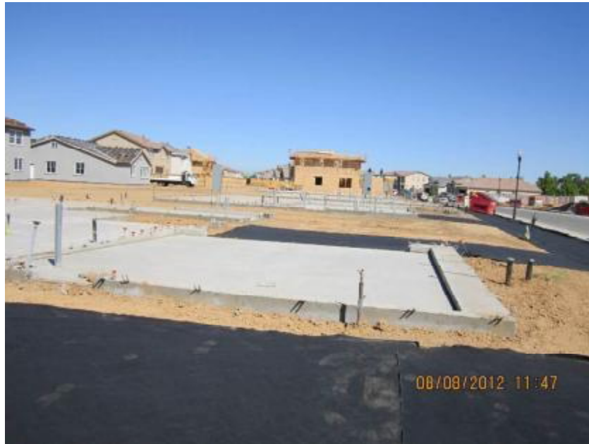
Photograph 1. View of lots with geotextile fabric applied around the perimeter of an active lot.
