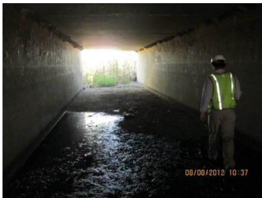
Photograph 2. View of box culvert access to outfall.
