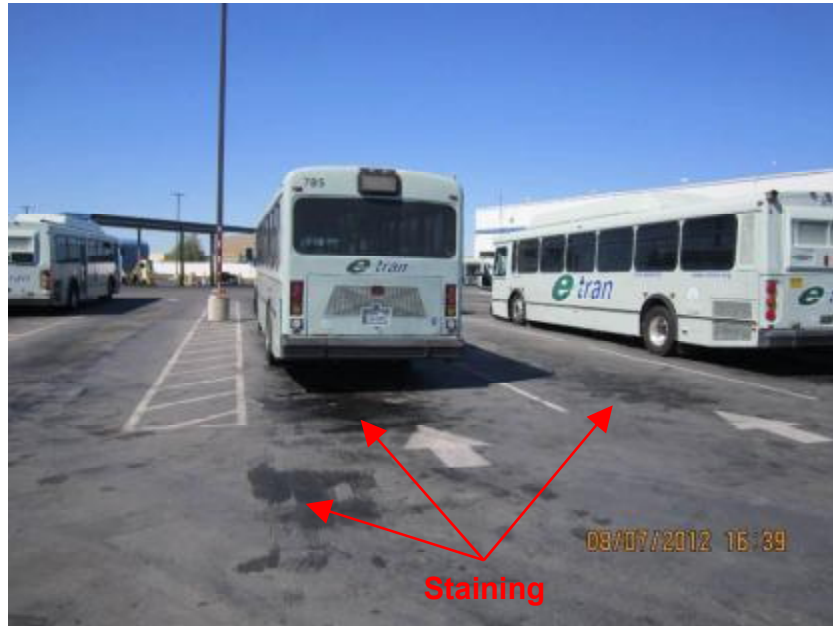
Photograph 9. Example of staining on impervious ground surface in bus storage and parking area.
