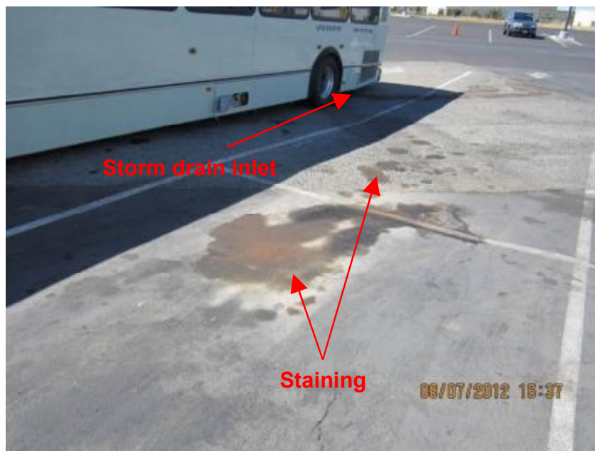
Photograph 8. View of staining on pervious and impervious ground surface upgradient of storm drain inlet shown in Photographs 6 and 7.
