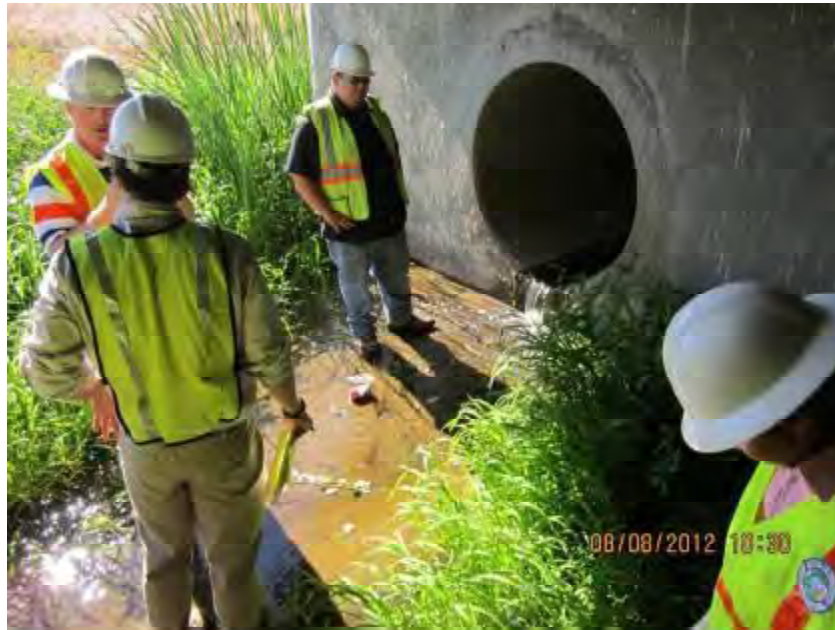
Photograph 3. View of outfall to Shed B Channel. Note dry weather flow from outfall.
