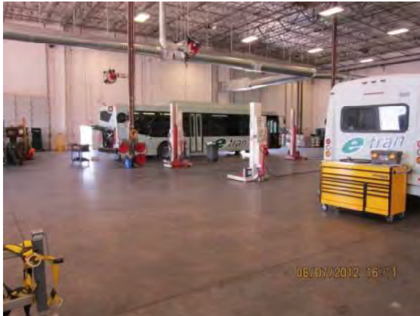
Photograph 1. View of portion of warehouse used for vehicle maintenance.
