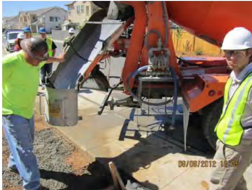
Photograph 5. View of contractor demonstrating how the “self-contained” cleaning procedure functioned on his concrete truck.
