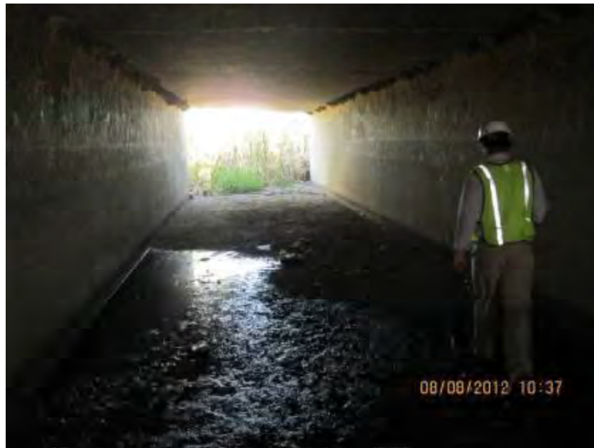
Photograph 2. View of box culvert access to outfall.
