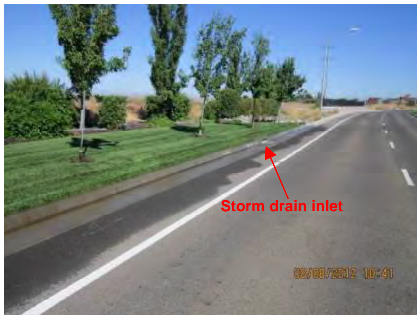
Photograph 5. View of turf area along roadway upgradient of outfall. Note evidence of irrigation flows to the curb and gutter.
