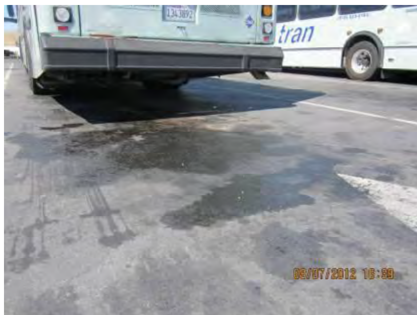
Photograph 10. Closer view of staining shown in Photograph 9.
