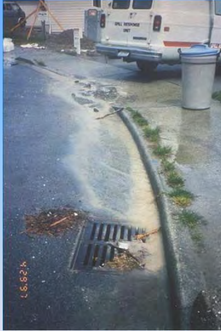
Illicit Discharge of Sediment Laden Water from Construction Site into Storm Drain Inlet
