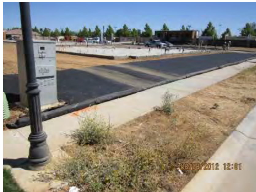
Photograph 2. View of area with geotextile coverage that was used for vehicle access.
