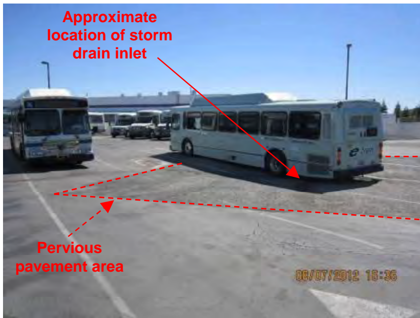
Photograph 6. View of bus parked over a storm drain inlet in an area of pervious pavement.
