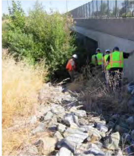
Photograph 1. View of access route to outfall.
