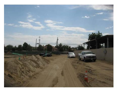
Photograph 1. View of southwest corner of the construction site. Note that the site had been initially graded and a contractor was installing building foundation pads at the time of the site visit.
