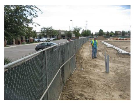
Photograph 2. View of the eastern perimeter of the construction site. Note that there is no silt fence to prevent sediment from leaving the site.
