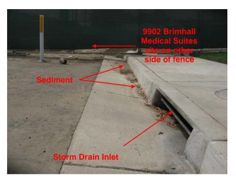
Photograph 3. The construction site lacked general erosion and sediment control measures (e.g., silt fence). View of storm drain inlet on roadway adjacent to the project near the southeast corner of the site. Note sediment in curb and gutter flow line and lack of inlet protection BMPs.
