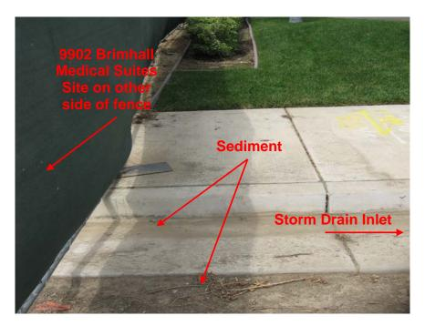
Photograph 4. Alternate view of sediment in curb and gutter flow line upgradient of unprotected storm drain inlet shown in Photograph 3. It was not clear to the EPA Inspection Team whether the drain inlet discharged to the City's MS4 or to a retention basin.
