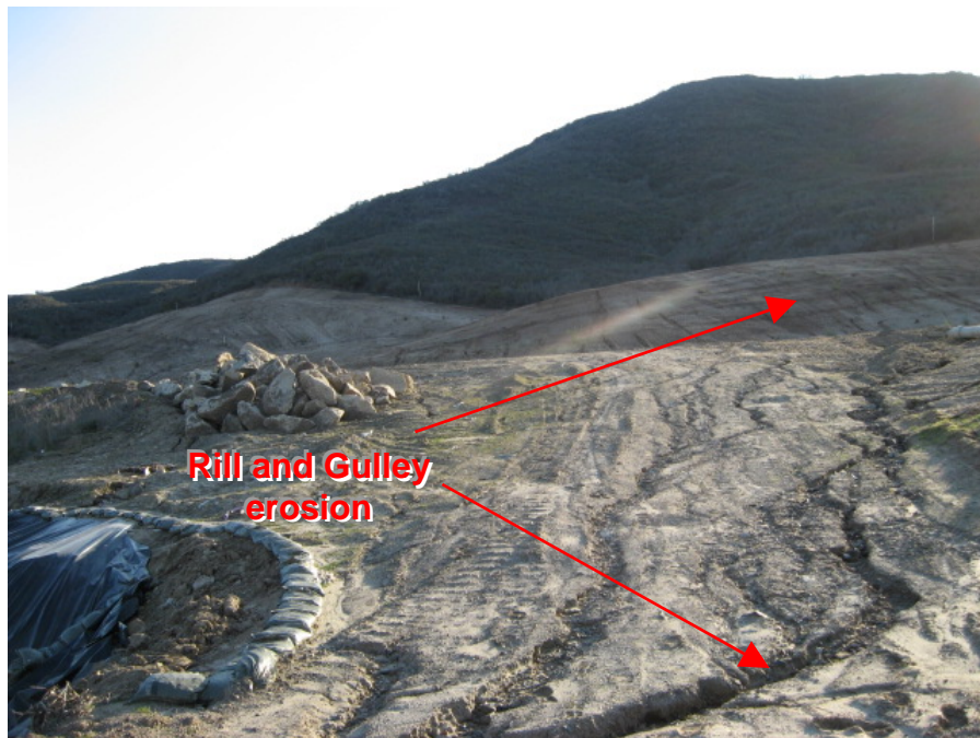
Photograph 6: Rill and gulley formations on the disturbed slope leading to the sediment trap BMP
