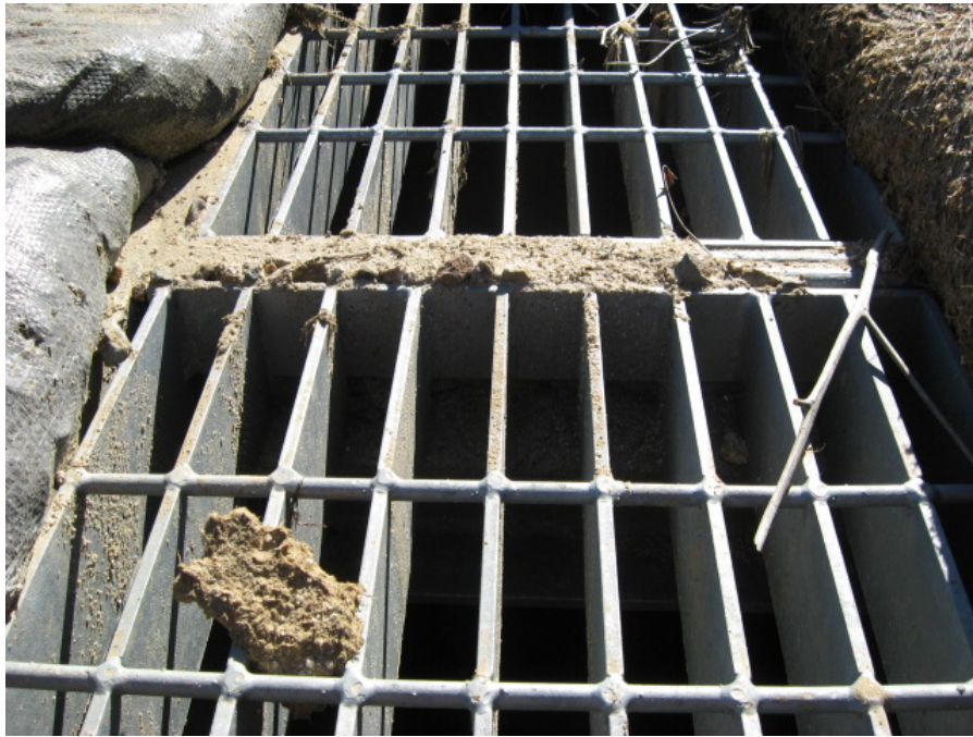
Photograph 11: Evidence of a previous failure event was observed, including sediment that had been discharged to a down-gradient storm drain inlet
