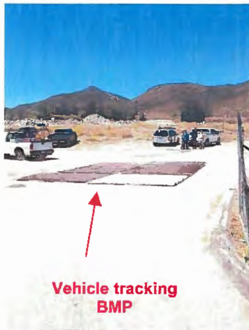
Photograph 1. Wendy Drive/101 Interchange Site Visit – View of a vehicle tracking BMP at the entrance to the material storage area.
