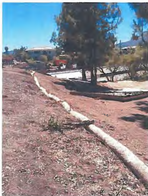
Photograph 5. Wendy Drive/101 Interchange Site Visit – View of fiber rolls installed along the slope of the embankment on the north side of Wendy Drive.
