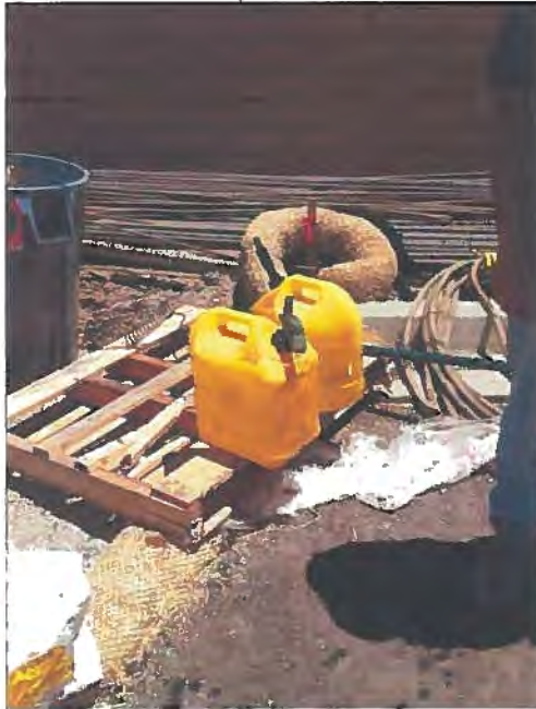
Photograph 5. Many Mansions Site Visit – View of gasoline container without secondary containment.
