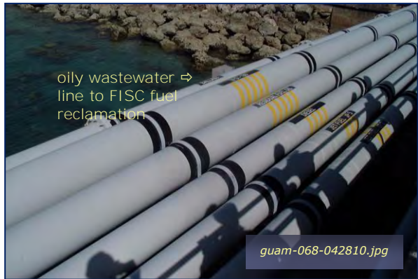
Photo #3-10: Fueling Piers - Bilge and Ballast Line Taken By: Greg V. Arthur Date: 04/28/10
