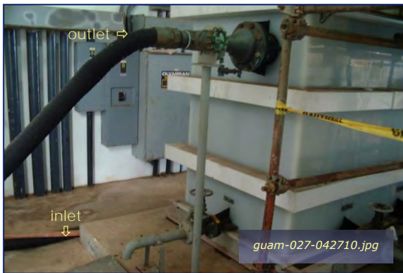
Photo #3-9: Papa Wharf - Bilge Oily Water Separator Taken By: Greg V. Arthur Date: 04/27/10
