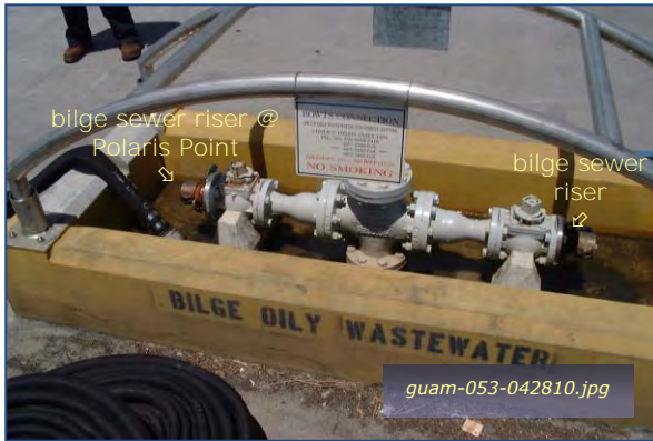
Photo #3-7: Bravo Wharf - Bilge Sewer Riser Taken By: Greg V. Arthur Date: 04/28/10
