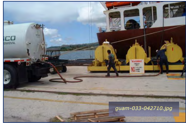
Photo #3-8: Lima Wharf - Bilge to Holding to Tanker Taken By: Greg V. Arthur Date: 04/27/10
