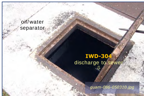
Photo #1-10: Bldg 18004 – Oil Water Separator Taken By: Greg V. Arthur Date: 05/03/10
