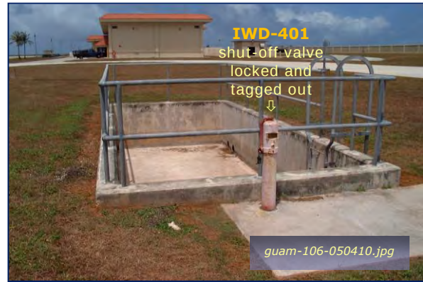
Photo #1-8: Satellite Fueling Station – Catchment Pit Taken By: Greg V. Arthur Date: 05/04/10
