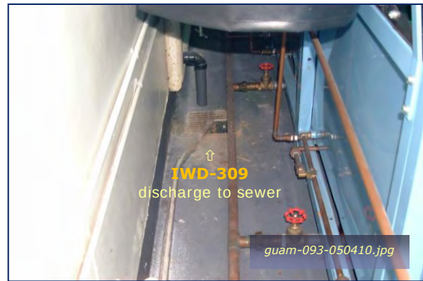
Photo #1-20: Bldg 17006 – NDT Discharge to Sewer Taken By: Greg V. Arthur Date: 05/04/10
