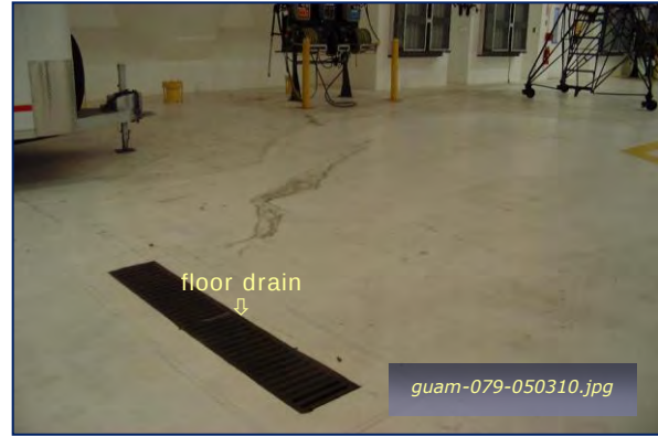
Photo #1-2: Hanger 2 - Floor Drain to O/W Sep Taken By: Greg V. Arthur Date: 05/03/10
