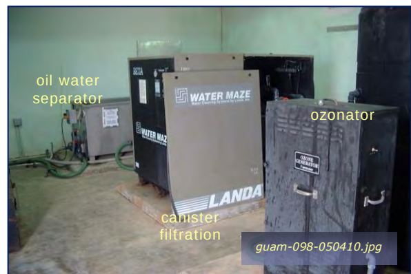
Photo #1-22: Bldg 2641 – Wash Rack Recycling Sys Taken By: Greg V. Arthur Date: 05/04/10
