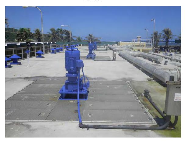
Picture 12: Drive motors for aerated digesters.
