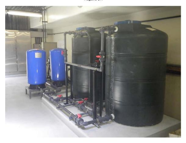
Picture 24: Dewatering polymer feed tanks.
