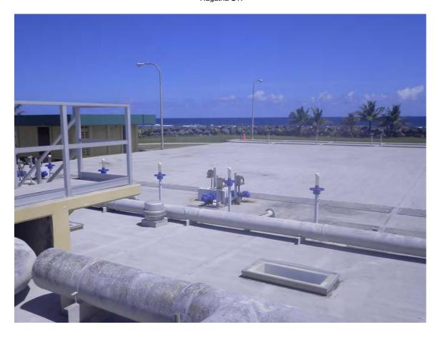
Picture 11: Collection ducts for odor control system at primary clarifiers.
