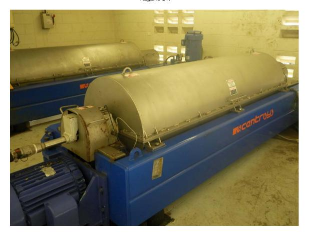
Picture 21: Dewatering centrifuges.
