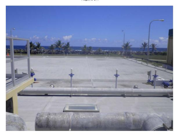
Picture 10: Concrete roof over primary clarifiers.
