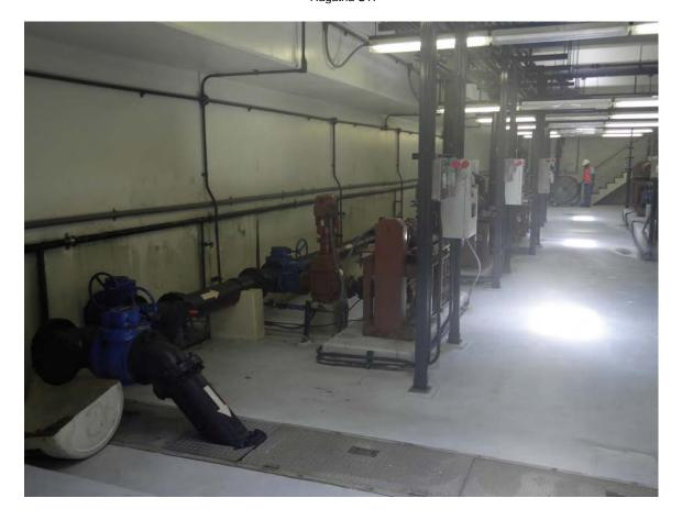
Picture 26: Grinders and sludge pumps for primary clarifiers.
