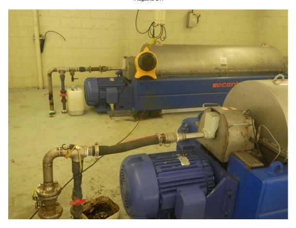
Picture 22: Feed lines for centrifuges.
