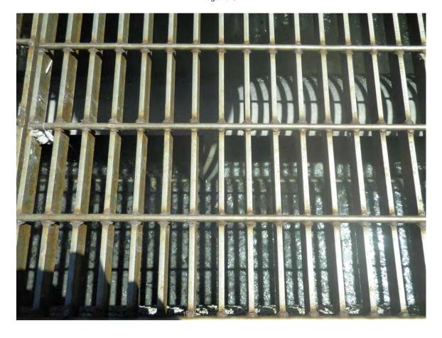
Picture 16: Surface skimmer trough for primary clarifier effluent
