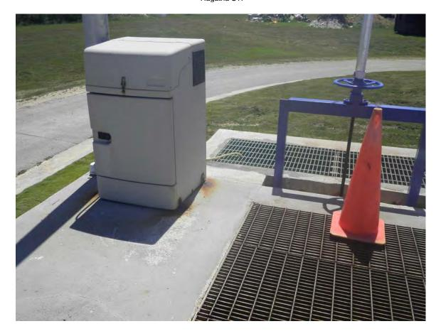
Picture 19: Effluent automatic sampler.
