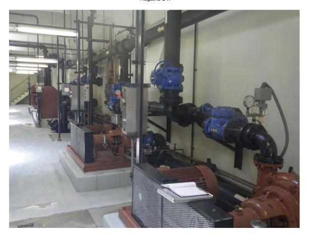
Picture 25: Sludge pumps for primary clarifiers.
