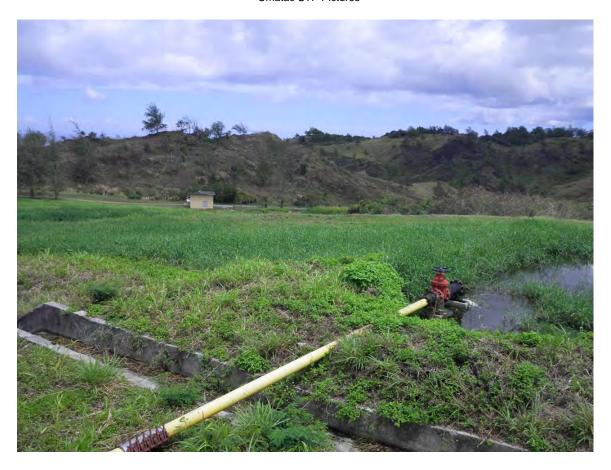
Picture 23: Looking down hill across Land Application Site A towards recirculation pond. Line in foreground is discharging water pumped from the recirculation pond by the pump station near upper left corner of photo.
