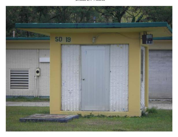
Picture 21: Pump Station 19 pumps effluent from the facultative lagoon to the recirculation pond.
