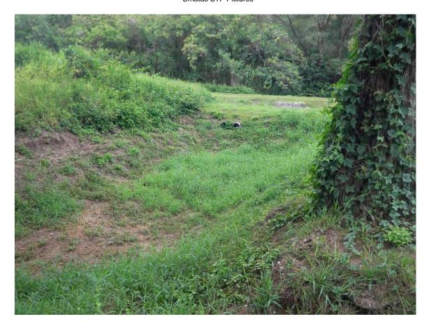
Picture 14: Discharge pipe in by-pass retention basin.
