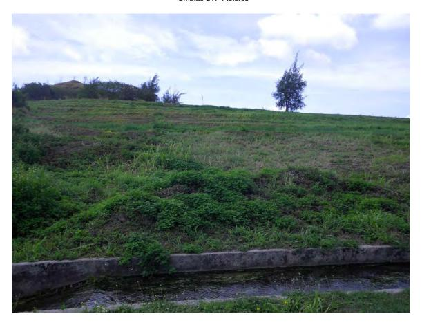
Picture 22: Looking up hill to Land Application Site A. Channel at bottom is returning runoff from land application sites back to recirculation pond.
