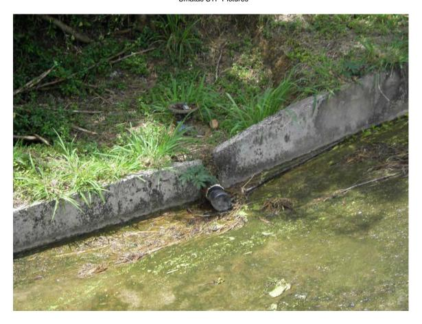
Picture 30: Valved and capped pond drain line.
