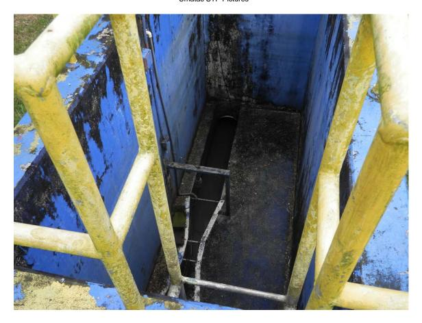
Picture 3: Unused Parshall flume for measuring influent flow rate. A depth monitoring device is installed in the pipe discharging into the flume at the top of the photo.
