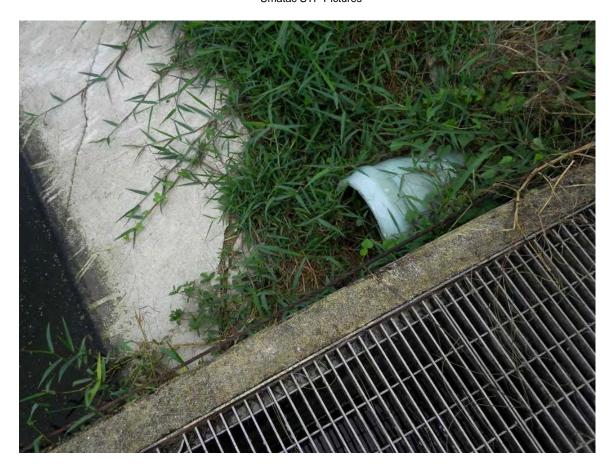
Picture 11: High level bypass pipe inlet for facultative pond.
