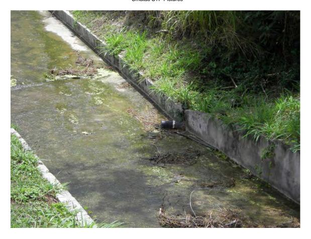
Picture 29: Capped line used to drain recirculation pond. Channel discharges to the Tocguan River. This location is downstream of the sample collection point.
