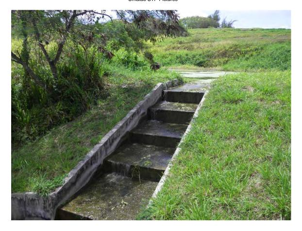
Picture 28: Recirculation pond overflow discharge to Tocguan River.
