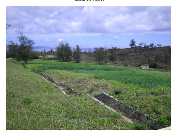
Picture 24: Runoff collection channel that returns excess water to recirculation pond.
