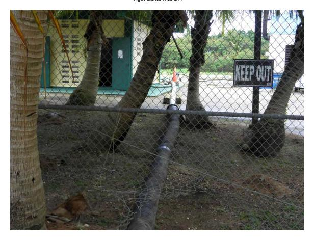
Picture 3: Discharge line from trailer mounted pump to contact basin.
