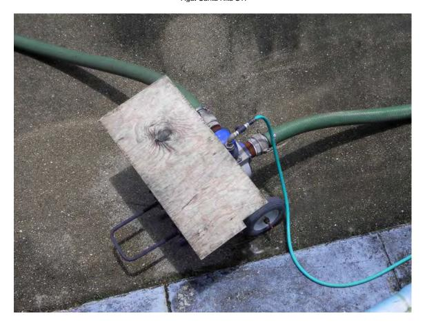
Picture 21: Portable pump used to pump waste solids from clarifier to sludge storage lagoons or tanker truck.
