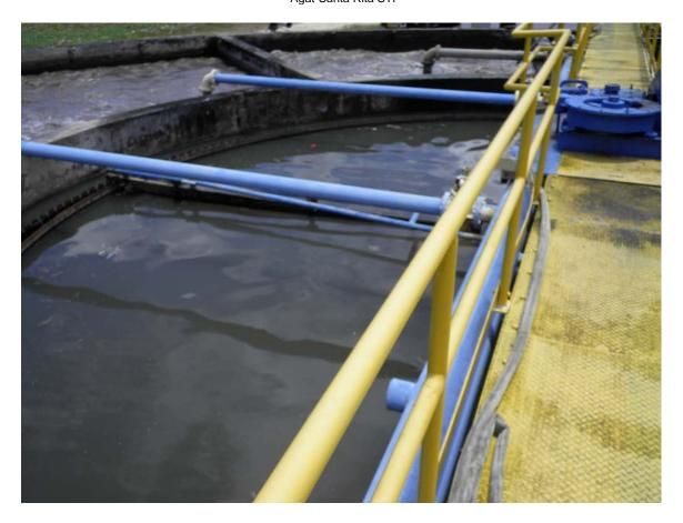
Picture 16: View across clarifier to digester. Blue lines are aeration lines to digester.
