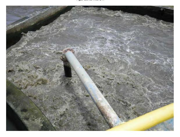
Picture 10: Air feed line for aeration system into contact tank.
