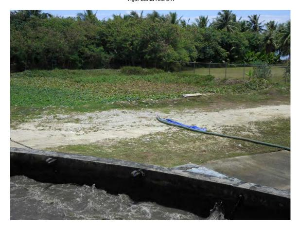
Picture 19: Sludge lagoon with line from portable sludge pump.
