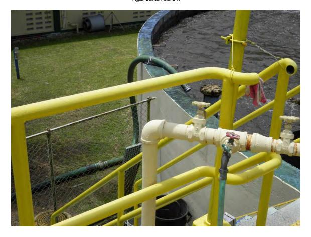
Picture 22: Intake for portable sludge pump over lip of digester.
