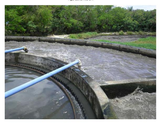
Picture 11: Stabilization tank. Blue lines are for aeration.
