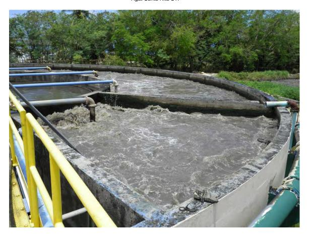
Picture 7: Contact tank. Pipe in far right is by-pass discharge line. Influent line on far left partially hidden by guard rail. Green line into basin near top is air line.
