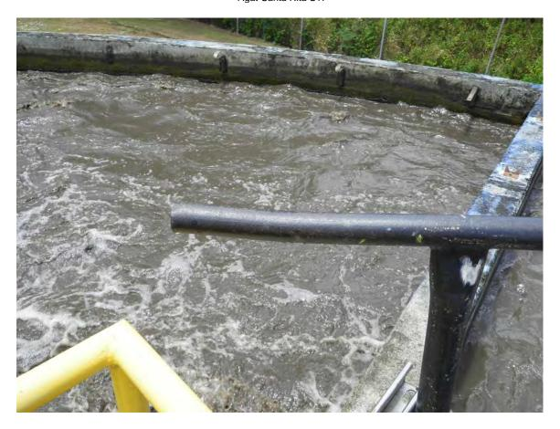
Picture 13: Baffle wall separating stabilization tank and contact tank. Hydraulic connection is through a port in the baffle wall to allow flow to pass between the tanks.
