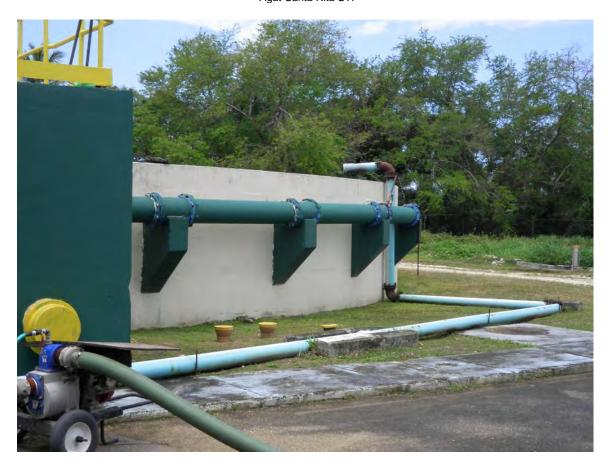
Picture 4: By-pass line into contact tank.
