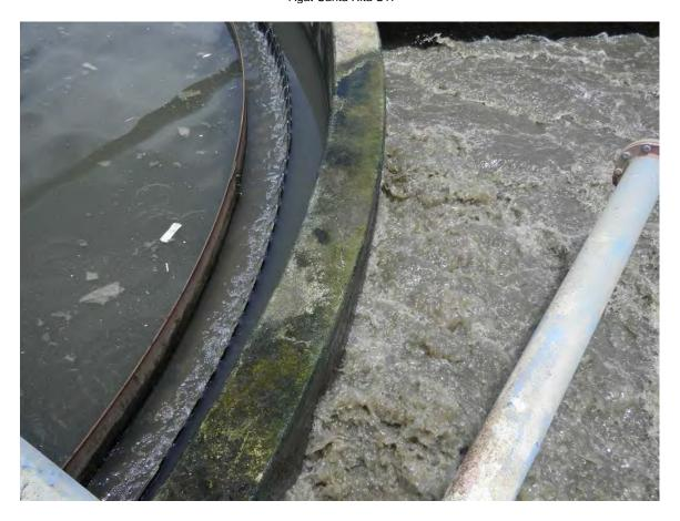
Picture 8: Concrete baffle wall separating contact tank from clarifier. Water was splashing over the wall into the discharge trough for the clarifier.
