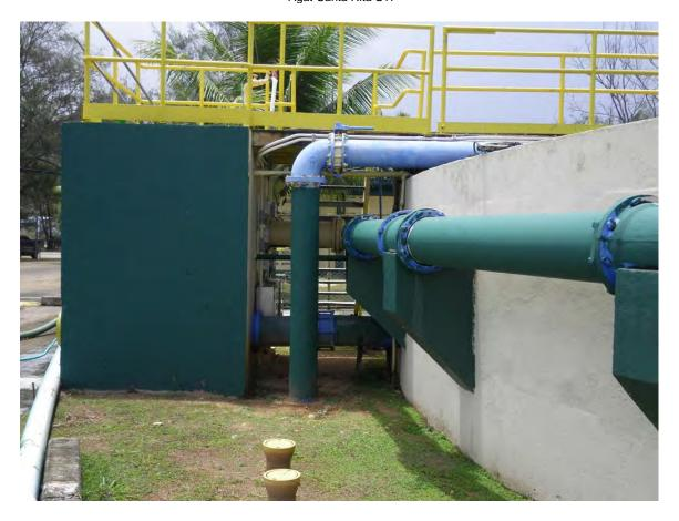
Picture 6: Blue line rising from ground is influent discharge into contact tank. Grey line running around tank is clarifier effluent to splitter box.
