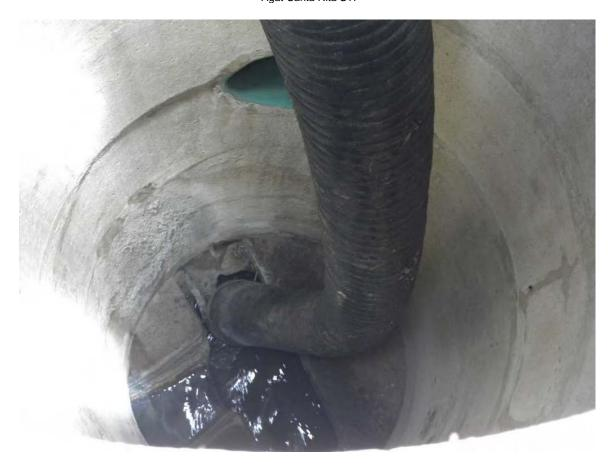
Picture 2: Intake line for trailer mounted pump used to by-pass head works.
