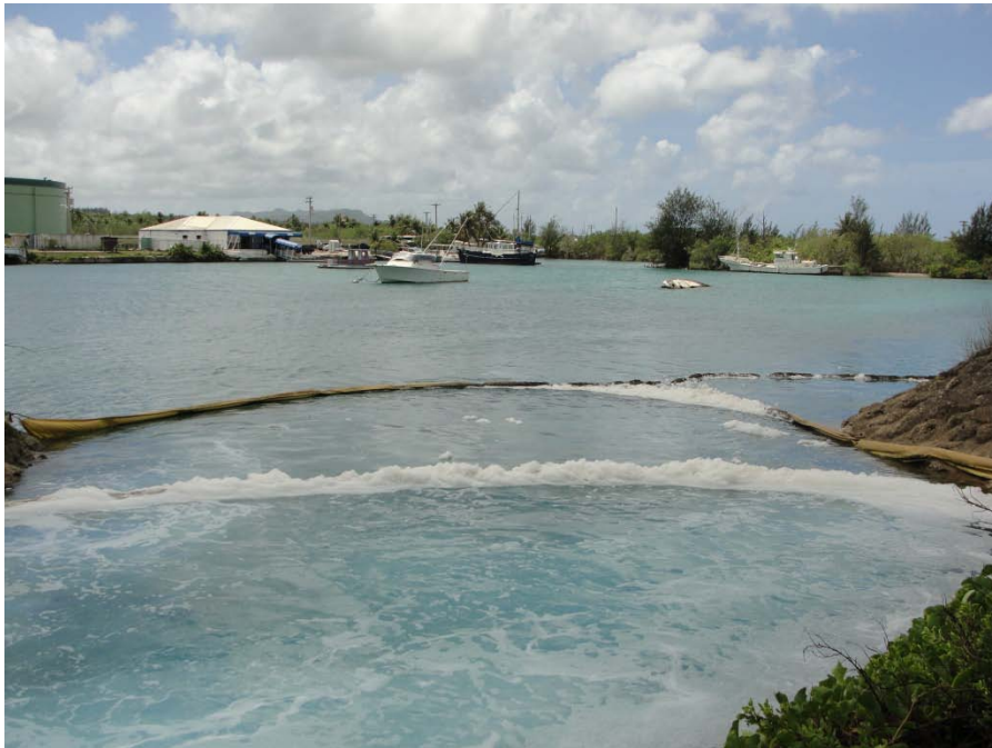
Photo 24: Receiving water at the mouth of the outfall structure.
