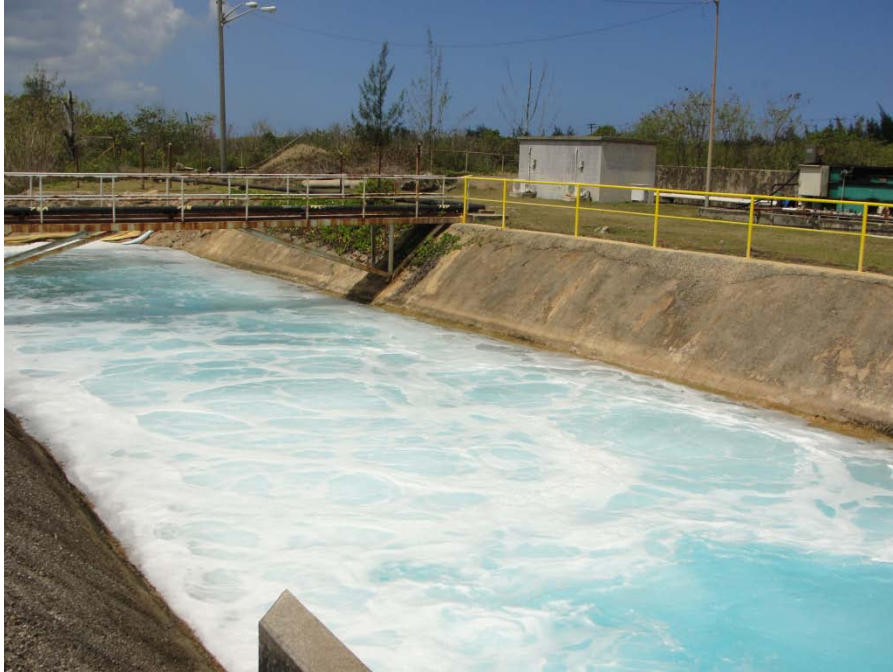
Photo 23: Outfall facing toward receiving water.
