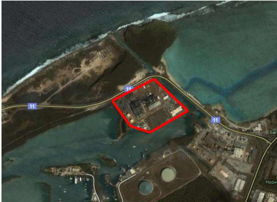
Photo 1: Overview of the Cabras Power Plant from Google Maps.
